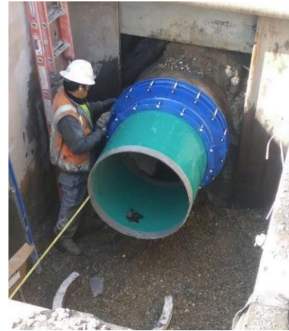
San Mateo Sanitary Sewer System
