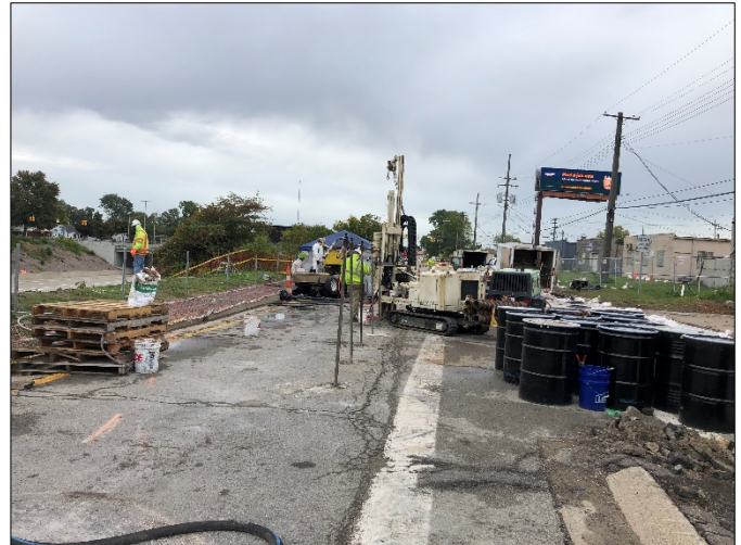
Groundwater treatment injections conducted in September 2020.
