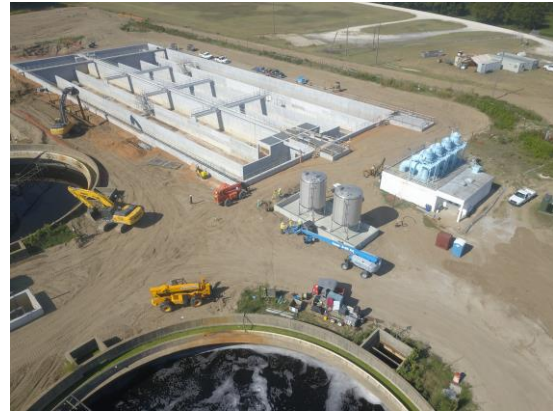
Disinfection Basin and Tank
