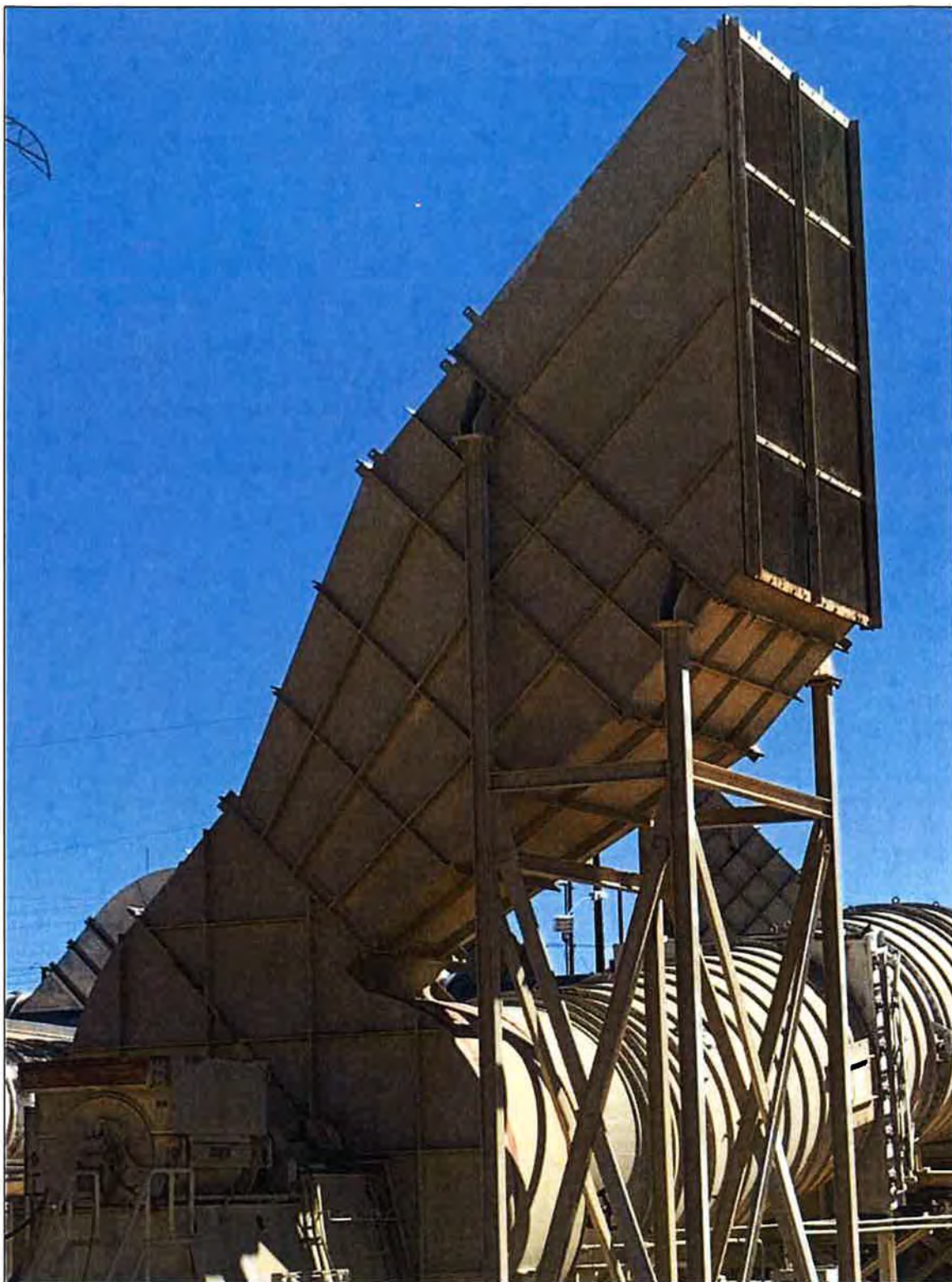
Figure 1 – Fan 700C Exhaust Shroud and Fan Screen
