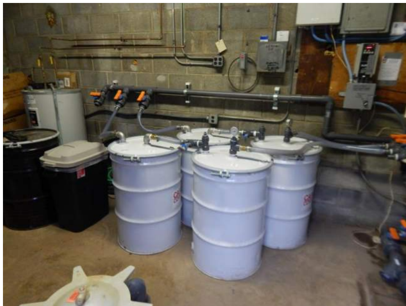
Carbon system showing carbon drums and effluent manifold.
