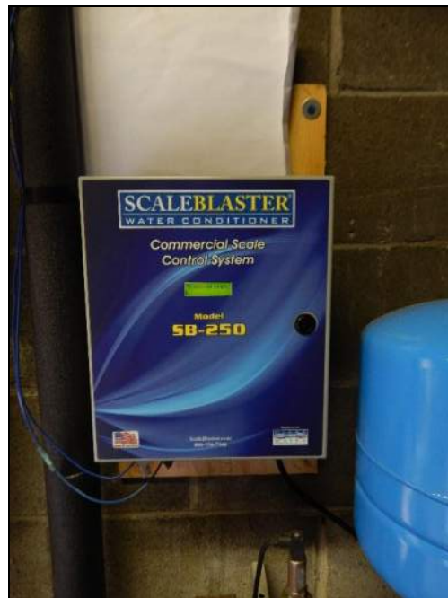
Electronic descaling system control box.
