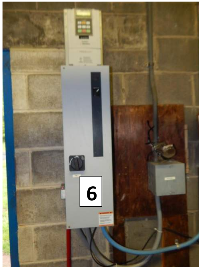
Variable Frequency Drive and shut off at well PW-6S. Formerly PW-5.
