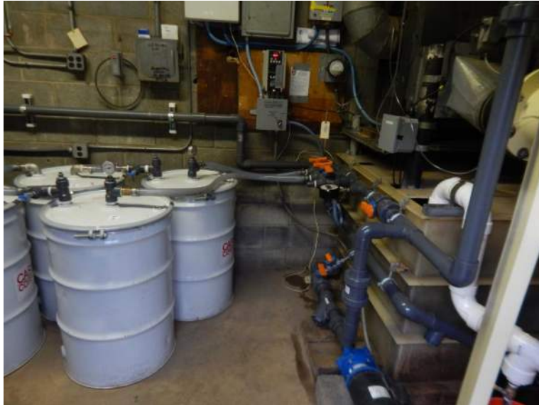
Carbon system showing influent manifold, pump, VFD, and carbon drums.
