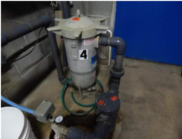
Filter and strainer system for well PW-4.
