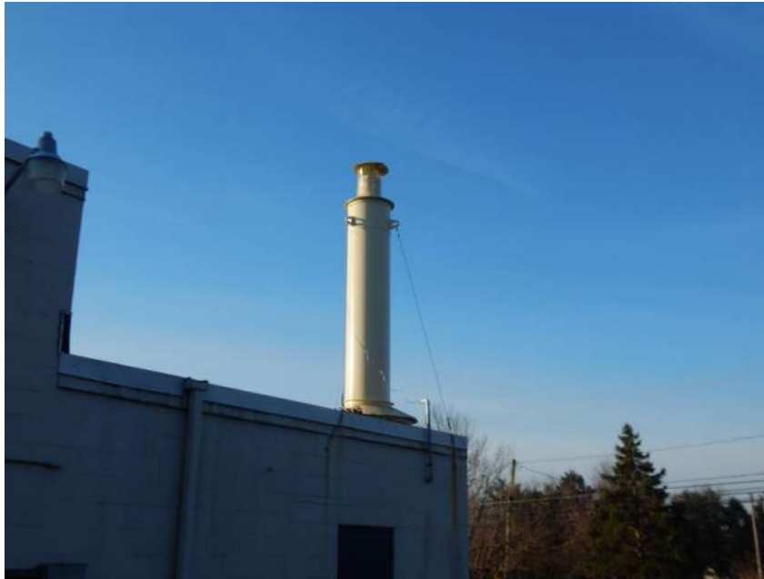
View of upper portion of air stripper.
