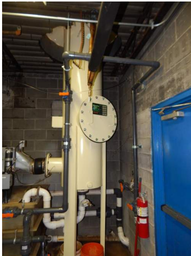
View of lower portion of air stripper tower.
