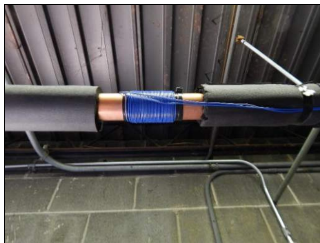
Wire coil for electronic descaler on 2-inch influent pipe.
