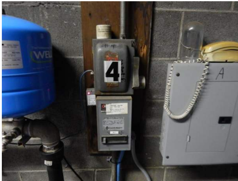
Shut off switch on well PW-4
