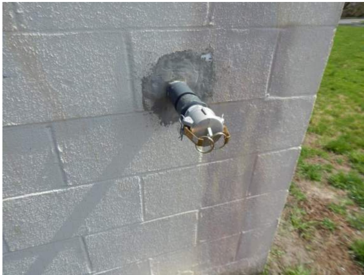
Exterior connection for introduction of investigation derived water into treatment system.
