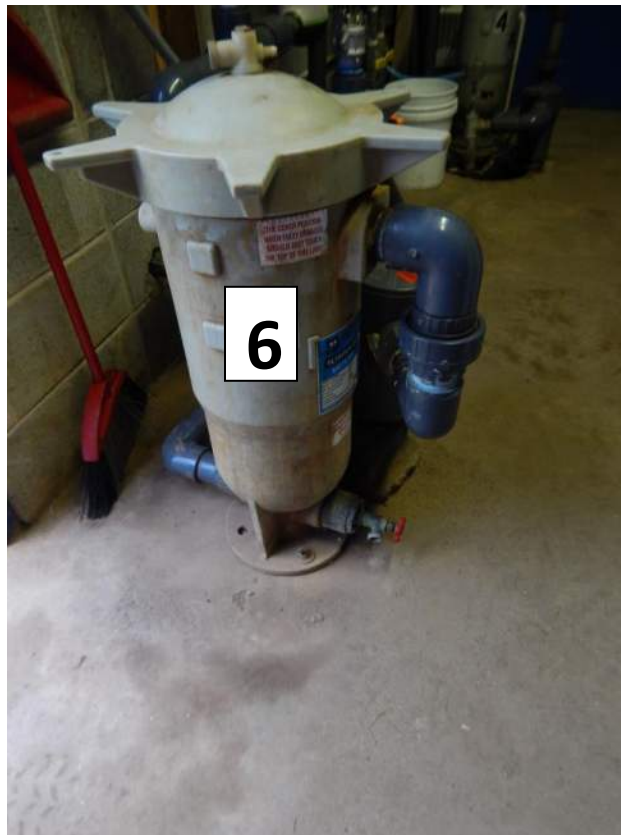
Filter housing for well PW-6S. PW-5 is no longer pumped, PW-6S has replaced this vessel and is labeled.
