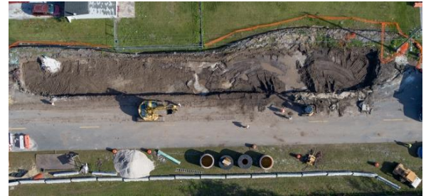
San Remo Road Construction
