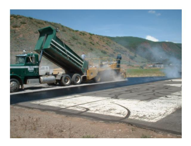
The validity of rubber-asphalt paving materials had been proven by our sister states of California and Arizona, which rely heavily on the process to provide a significant increase in the longevity of the pavement and the wise recycling of used auto tire products. Reflective cracking has all but been eliminated with this process and the pavement remains flexible and viable long after non-rubberized materials have failed.
