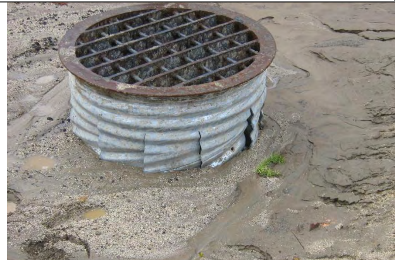
Photograph 12 – Close-up view of sediment basin No. 1 outlet structure with sediment accumulation
