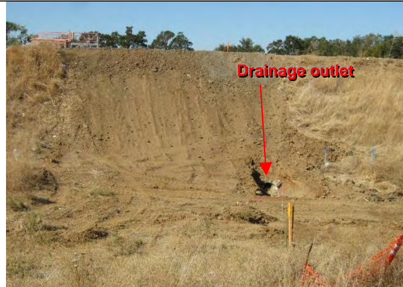
Photograph 6 – Drainage outlet below unstabilized embankment slope adjacent to the highway.
