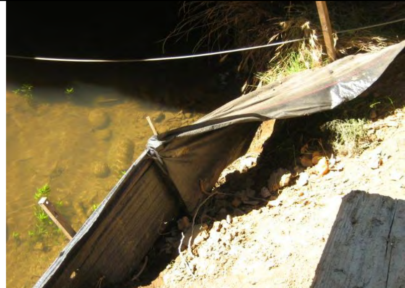
Photograph 24 – Silt Fence not properly entrenched to retain sediment adjacent to Yankee Slough waterway
