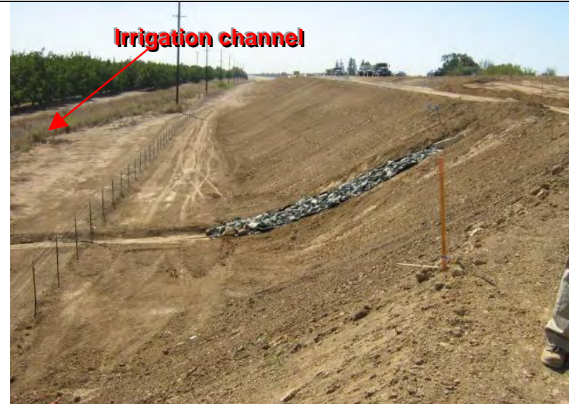
Photograph 26 – Large expanse of disturbed slope area with only rock and no perimeter BMPs.
