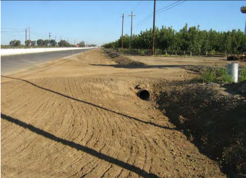
Photograph 1 – Drainage swale adjacent to roadway without adequate BMPs implemented (Drill seeding only)
