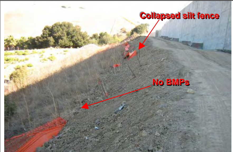
Photograph 6 – Fill slope along access road without BMPs
