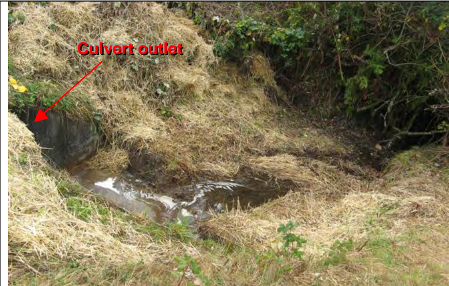
Photograph 6 – West side of culvert outlet (Note: Straw around and within drainage channel)
