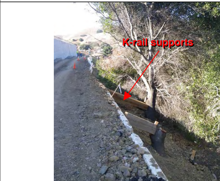
Photograph 4 – Failed area along access road
