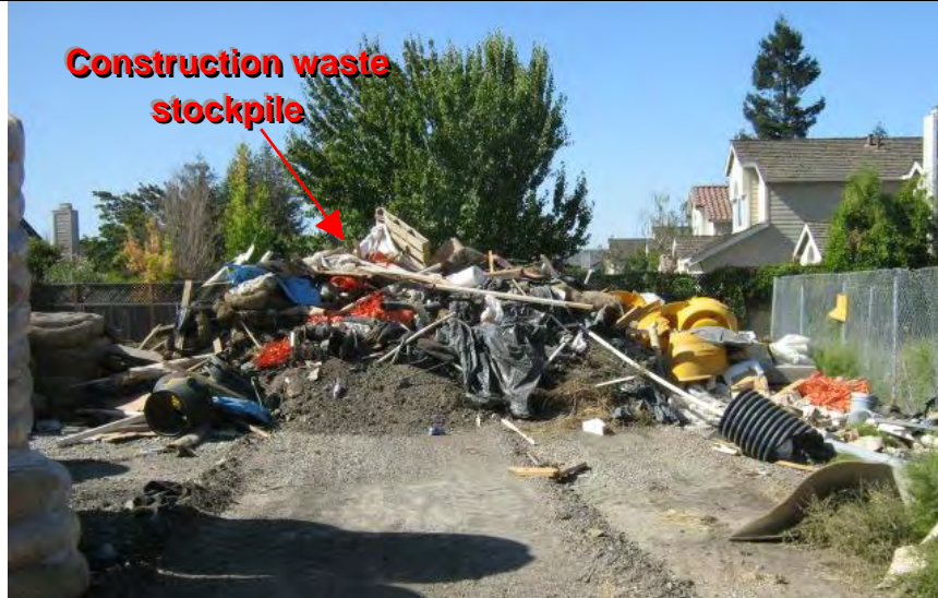
Photograph 5— Uncovered and uncontained construction waste
