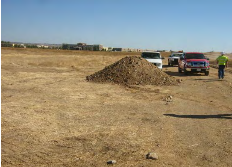
Photograph 9 – No BMPs implemented for stockpile management near the North Ingram Slough bridge crossing
