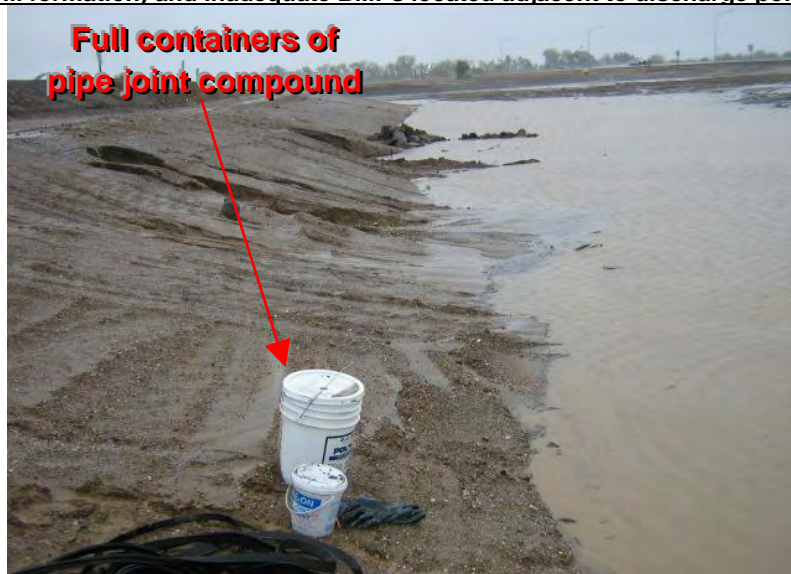
Photograph 7—Pipe joint compound located in the eastern sediment basin
