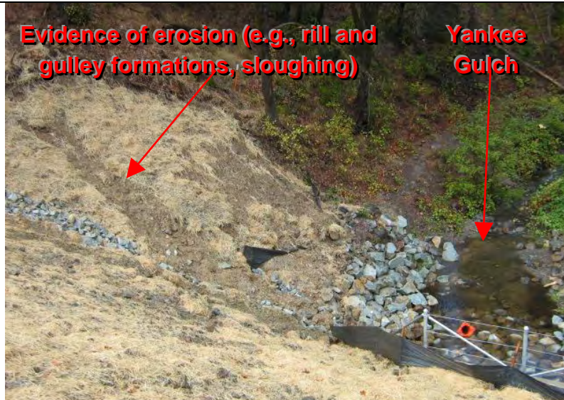
Photograph 9— Evidence of erosion (e.g., rill and gulley formation) and sediment transport from the disturbed slope failure
