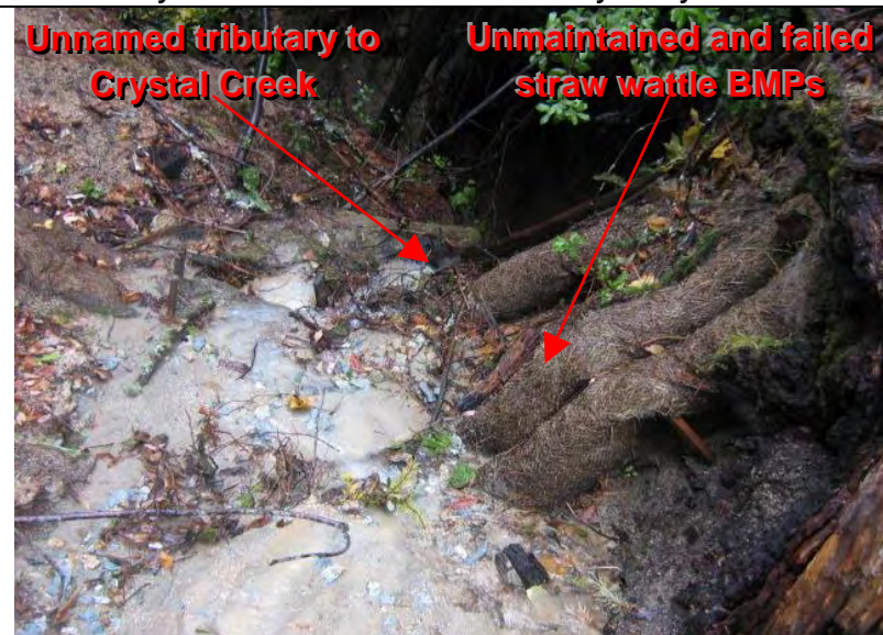
Photograph 8 – Visible evidence of the discharge of sediment to the unnamed tributary to Crystal Creek, and failed straw wattle BMPs observed
