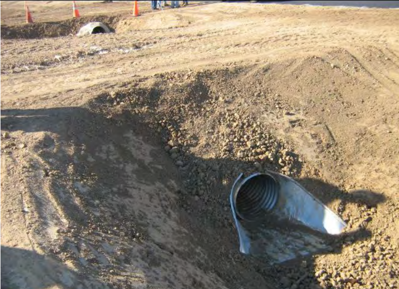
Photograph 7 – Culvert pipe inlet with no BMPs implemented – drains to irrigation ditch.
