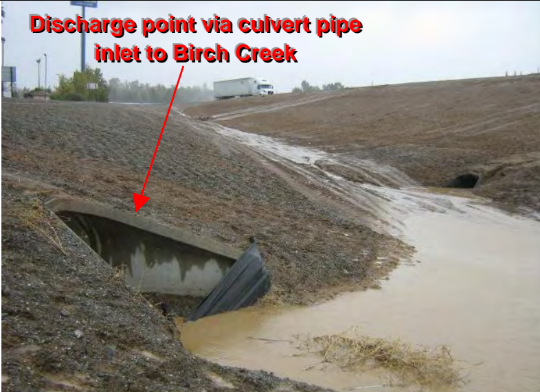
Photograph 9—Discharge point, culvert inlet and drainage pipe leading to Birch Creek
