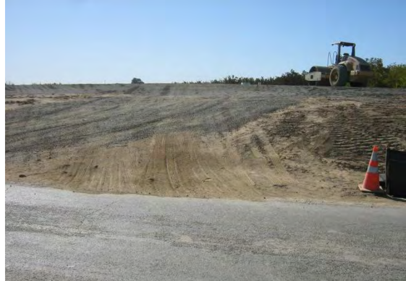
Photograph 20 – Adequate tracking control BMPs had not been implemented at the Wilson Road intersection.
