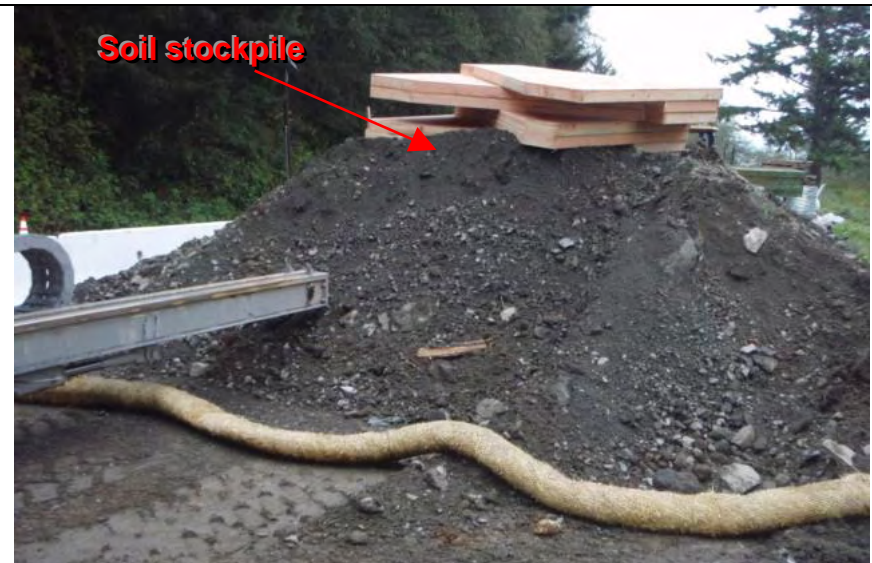
Photograph 14— Another example of straw wattle not staked or entrenched into ground. Inappropriate application of wattles on impervious surface.
