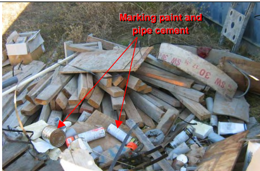
Photograph 3 – Construction wastes and chemicals improperly disposed
