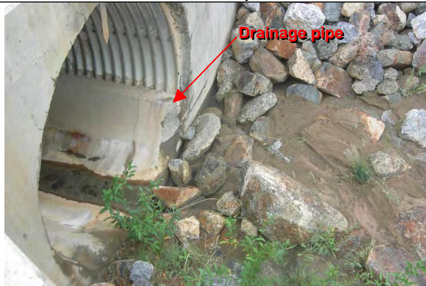
Photograph 7 – Sediment accumulation at down-gradient drainage pipe inlet
