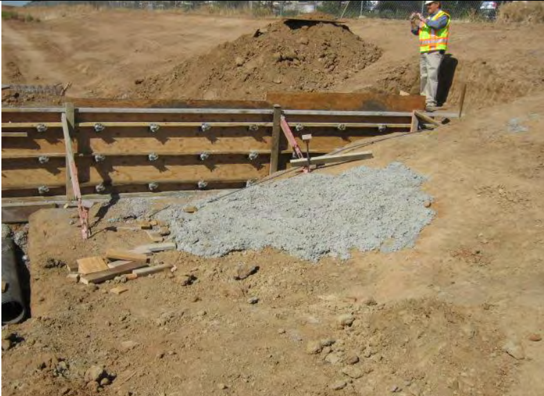
Photograph 1 – Improper concrete waste disposal practices
