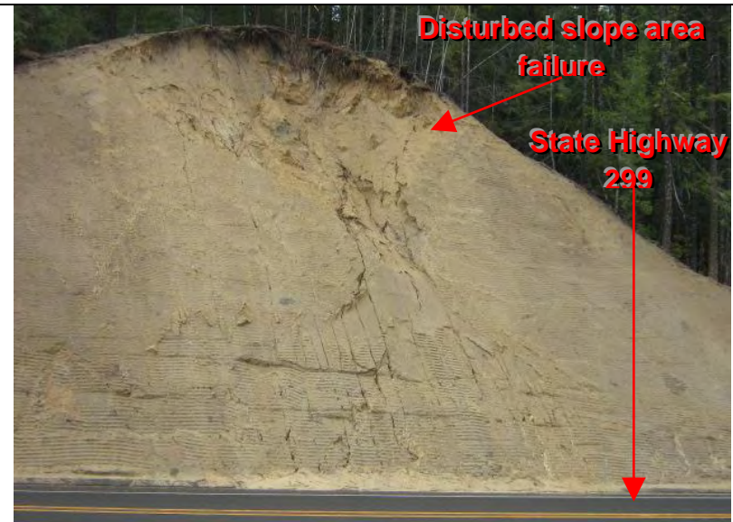
Photographs 18 – Adequate BMPs were not implemented to prevent the discharge of sediment from a disturbed cut slope area adjacent to State Highway 299.
