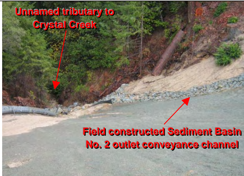
Photograph 5— View of sediment basin No. 2 outlet conveyance channel and confluence with the unnamed tributary to Crystal Creek
