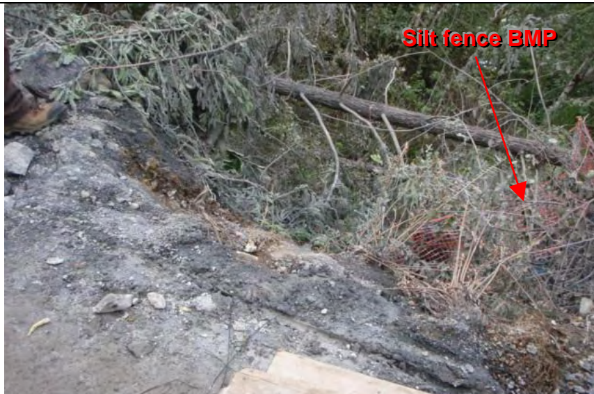
Photograph 7— Another example of silt fence BMP partially covered by collapsed vegetation - view down slope to silt fence BMP
