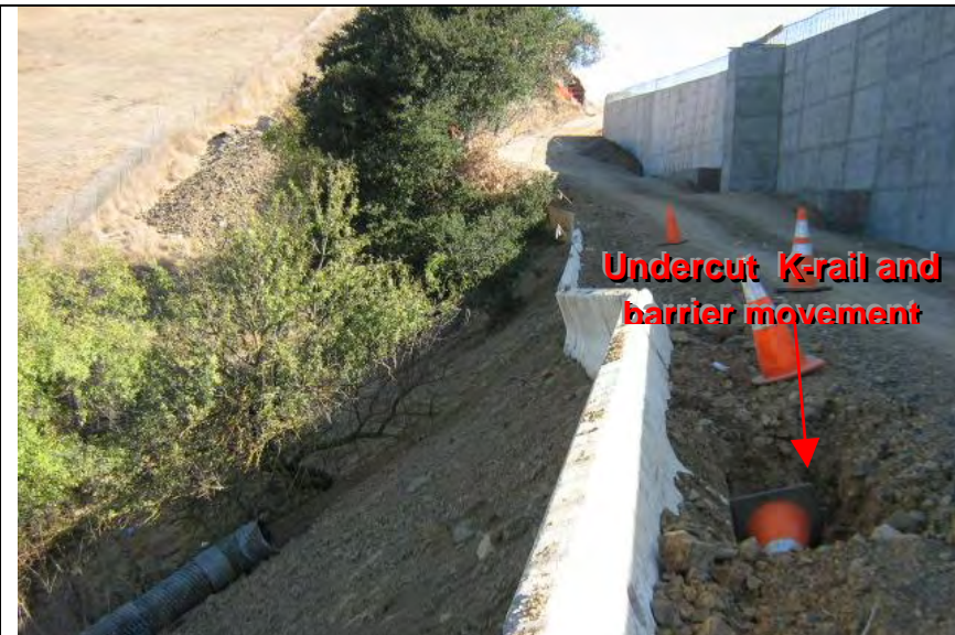
Photograph 2 – Failed fill slope along access road
