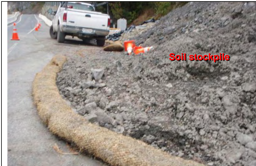
Photograph 13— Straw wattle not staked or entrenched into ground. Inappropriate application of wattles on impervious surface
