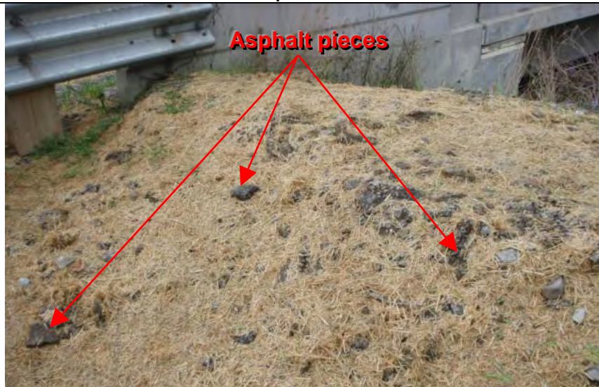
Photograph 11— Sidecast asphalt pieces along side of roadway at northern end of construction project
