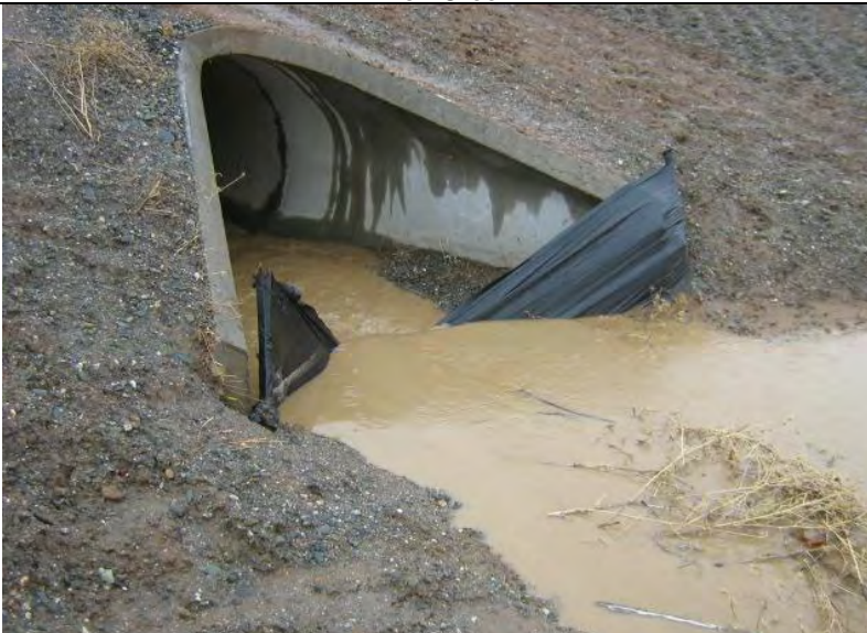
Photograph 11— Collapsed silt fence BMP and discharge of sediment laden runoff
