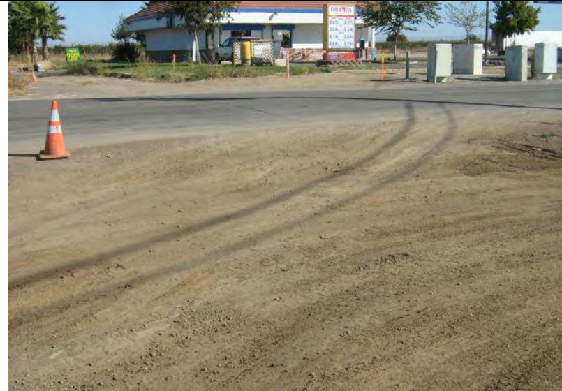
Photograph 12 – No tracking control BMPs implemented at Sta. 346 + 70.
