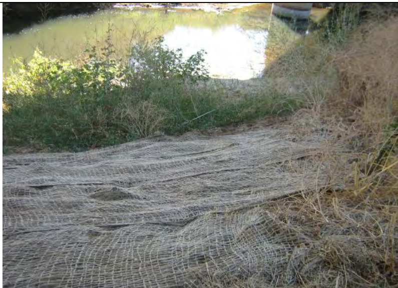
Photograph 1 – Erosion control blanket not properly installed (e.g., improper overlap – not shingled downgradient) adj. to Bear River at top.
