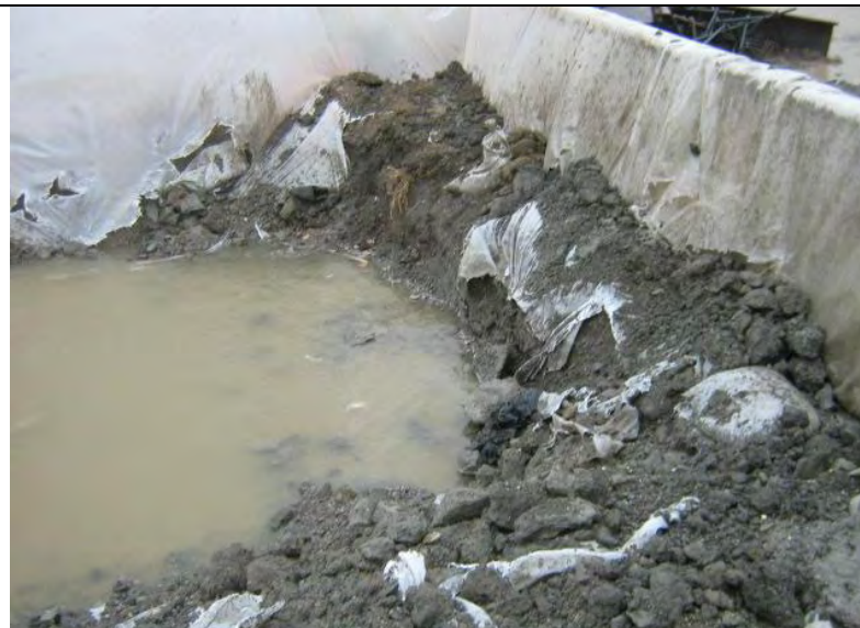
Photograph 2 – Close-up view of unmaintained (e.g., torn and deteriorated) concrete washout plastic liner
