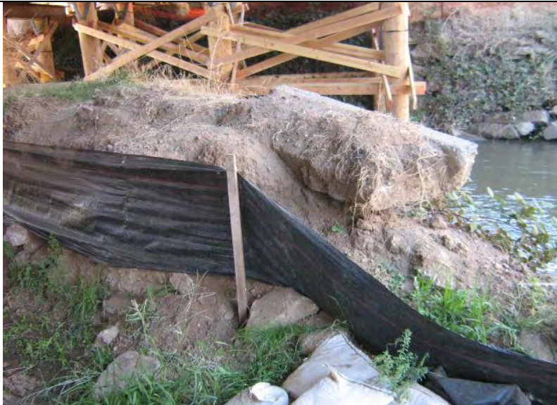
Photograph 11 – Silt Fence BMPs not properly installed (e.g., not entrenched) or maintained (e.g., collapsed) adjacent to Auburn Ravine
