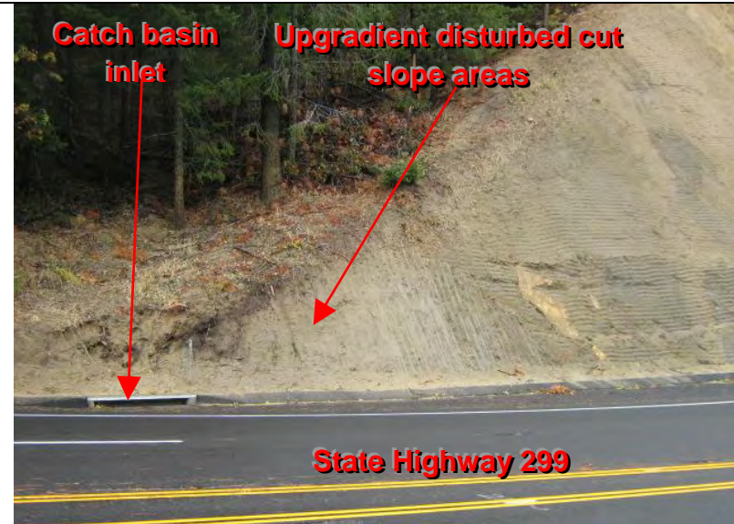
Photographs 22 – BMPs were not implemented to prevent the discharge of sediment from upgradient disturbed cut slope areas to catch basin inlets.
