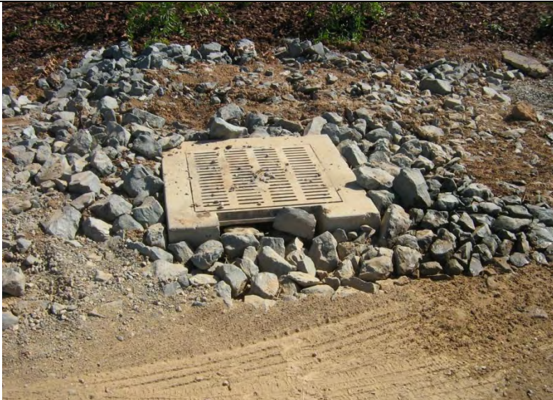
Photograph 17 – Close-up of Photograph 16. Adequate inlet protection had not been implemented.
