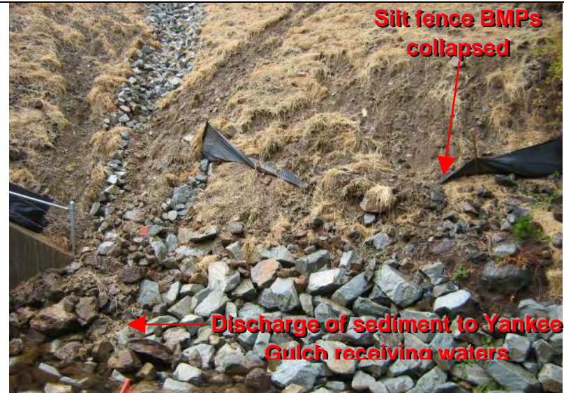
Photograph 10 – Silt fence BMPs collapsed in areas and evidence of the discharge of sediment to Yankee Gulch
