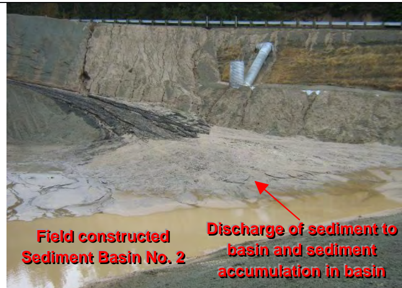
Photograph 2 – Discharge of sediment from disturbed slope area to field constructed sediment basin and sediment accumulation in the basin
