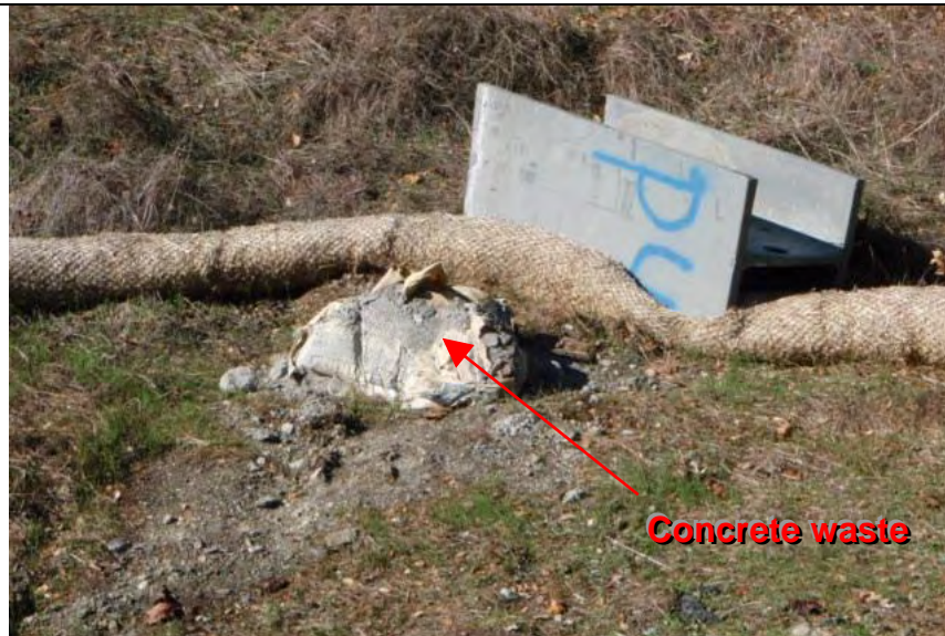
Photograph 11— Concrete waste near concrete waste container in staging area (Note: Straw wattle BMP not staked or entrenched into ground)
