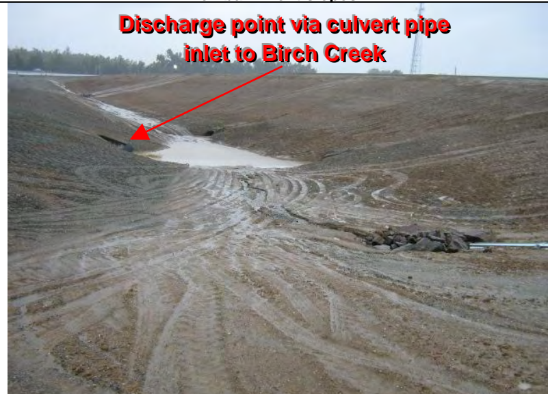
Photograph 4 – Adequate BMPs had not been implemented to prevent the discharge of sediment to the culvert inlet/drainage pipe leading to Birch Cr.
