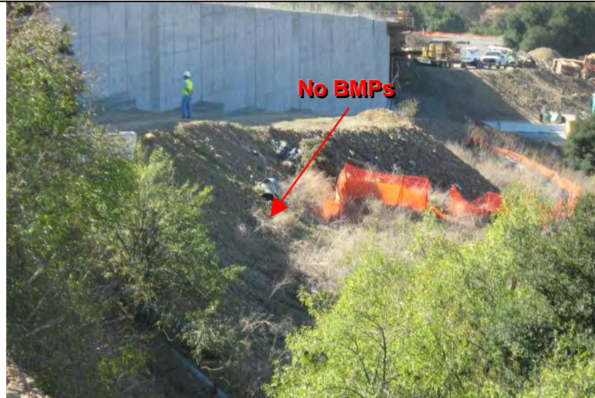
Photograph 5— Fill slope along access road without BMPs
