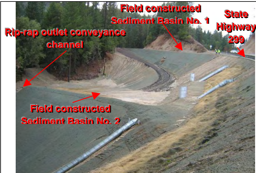
Photograph 9—Vantage point photograph depicting location of field constructed sediment basins No. 1 and No. 2 and their outlet.
