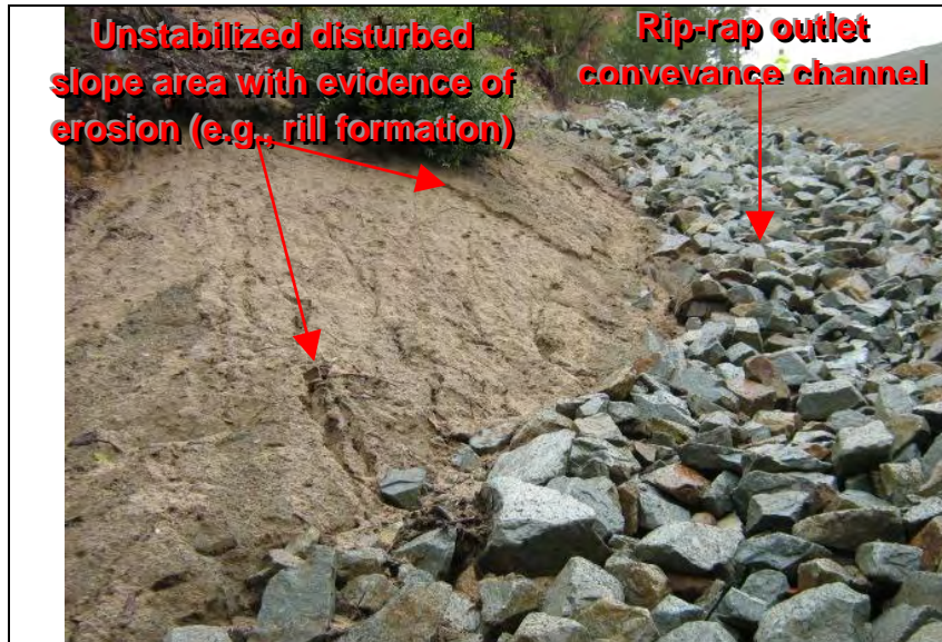
Photograph 17—Adequate BMPs were not implemented to prevent the discharge of sediment from disturbed slope area adjacent to the rip-rap conveyance channel which drains to the unnamed tributary.
