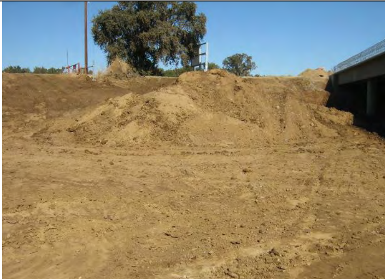
Photograph 5 – Soil stockpile with no perimeter controls or temporary stabilization located just upgradient of Bear River crossing.
