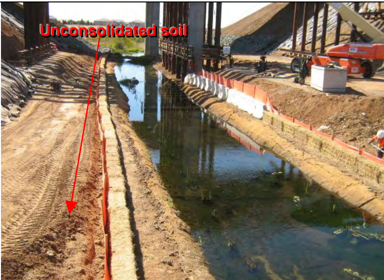
Photograph 3 – Unconsolidated soil placed between the toe of the slope and the perimeter control BMPs along the waterway
