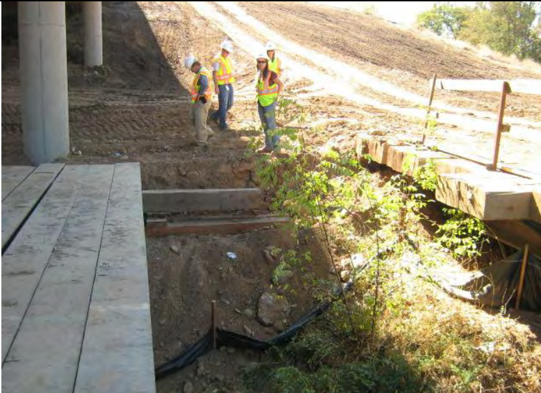
Photograph 23 – Silt Fence collapsed in areas and not properly maintained. Note large unstabilized slope area upgradient.
