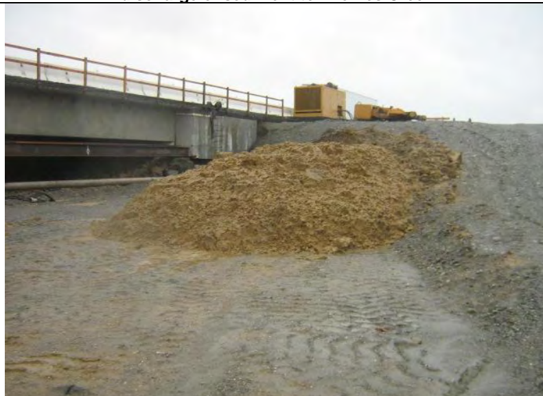
Photograph 11— Soil stockpile without BMPs
