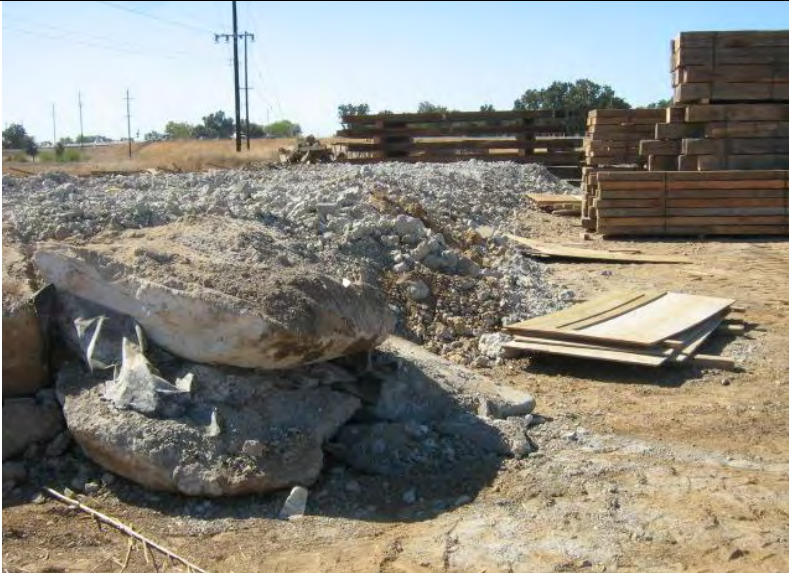
Photograph 9 – Uncontrolled/uncontained concrete waste
