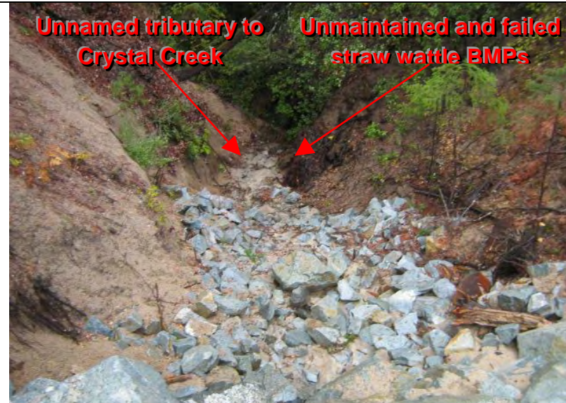
Photograph 6 – Close-up view of sediment basin No. 2 rip-rap outlet conveyance channel to unnamed tributary to Crystal Creek
