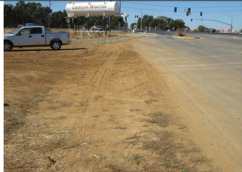
Photograph 12 – Tracking control BMPs not implemented for disturbed area of contractor parking. Observed sediment transport to roadway
