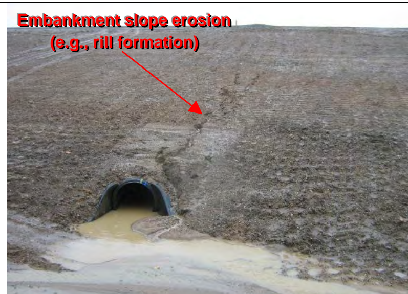
Photograph 6 – Embankment slope erosion (e.g., rill formation)
