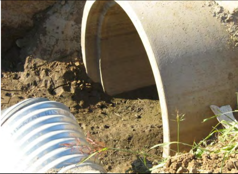
Photograph 9 – Visible sediment accumulation in the irrigation channel and associated culvert pipe
