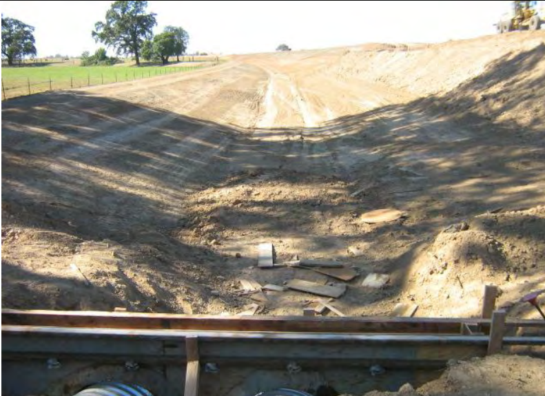
Photograph 17 – Upgradient areas of disturbance associated with pollution prevention BMP unstabilized. Drains to Auburn Ravine.
