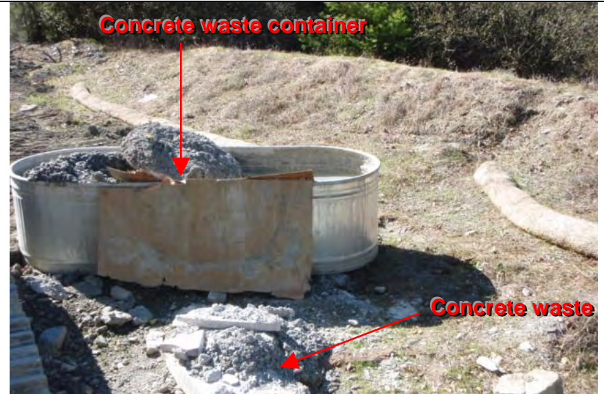
Photograph 10— Concrete waste and container in staging area (Note: Straw wattle BMP not staked or entrenched into ground)
