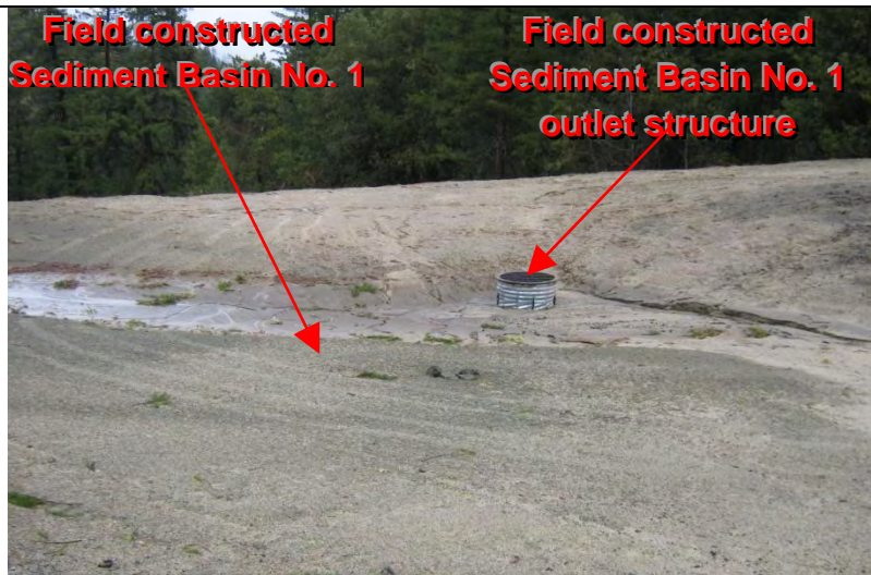
Photograph 11—Evidence of the discharge of sediment to and accumulated in the basin No. 1 which subsequently flows to basin No. 2 and the unnamed tributary to Crystal Creek
