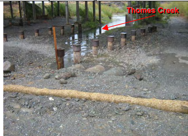
Photograph 8 – Erosion log BMPs were not adequately installed (e.g., not properly staked) adjacent to the flowing Thomes Creek
