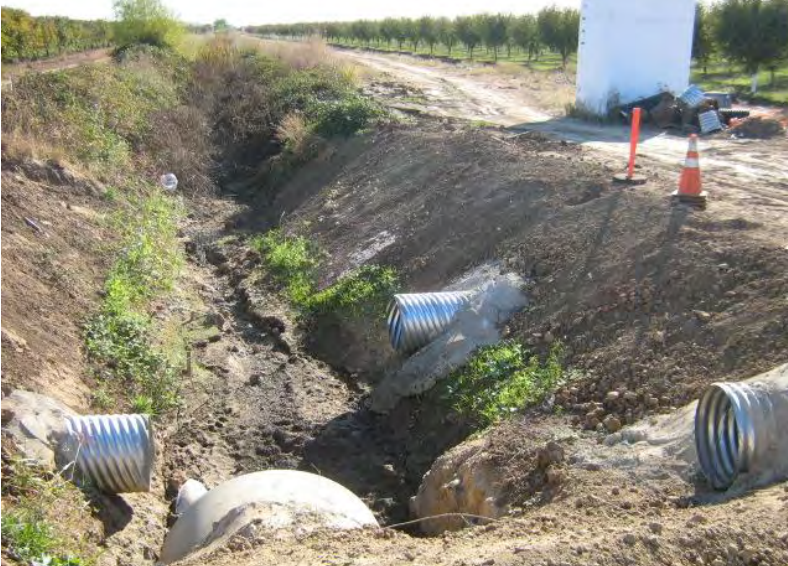
Photograph 5 – View looking upgradient on irrigation channel located adjacent to project. Note unstabilized slopes adj. to irrigation channel.
