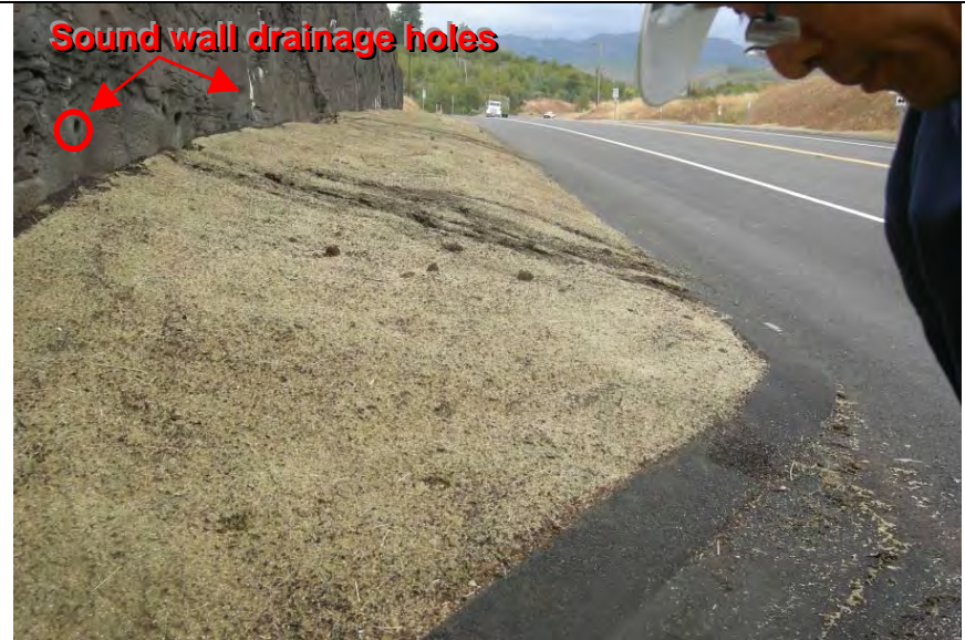
Photograph 2 – Run-off causing erosion along the highway shoulder
