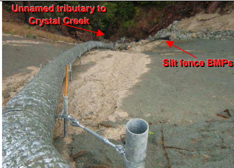
Photograph 13—Adequate BMPs were not implemented to prevent the discharge of sediment from upgradient disturbed slope areas
