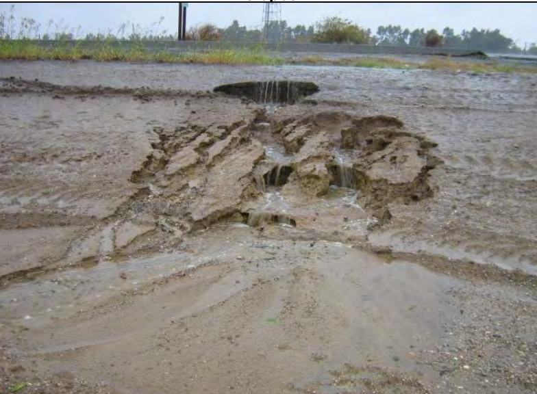
Photograph 3 – Sediment basin embankment slope erosion (e.g., gulley formation) and failure
