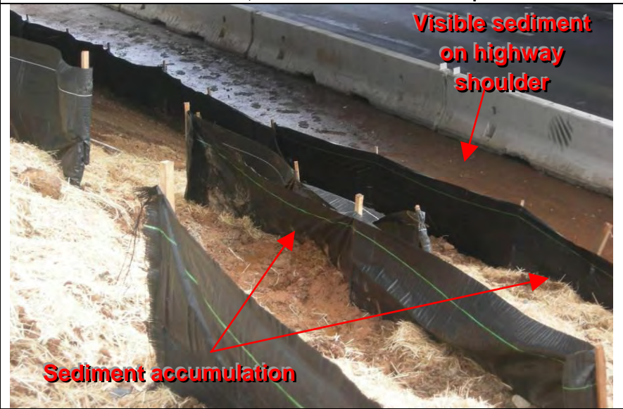
Photograph 4 – Silt fence on the north side of I-5, view facing south-southeast
