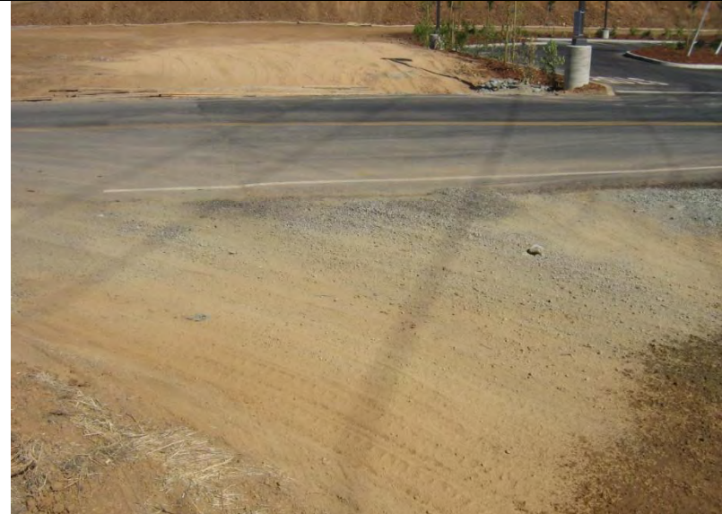
Photograph 10 – Tracking control BMPs not adequately maintained (e.g., sediment in rock pad and rock sparse in areas)
