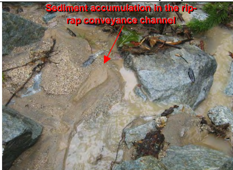
Photograph 7—Visible evidence of sediment accumulation in the rip-rap outlet conveyance channel which drains to the unnamed tributary
