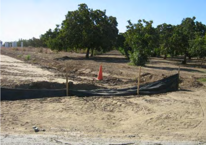
Photograph 19 – Silt fence not adequately maintained (e.g., collapsed in areas) near the new Hwy 99 and Wilson Road intersection.
