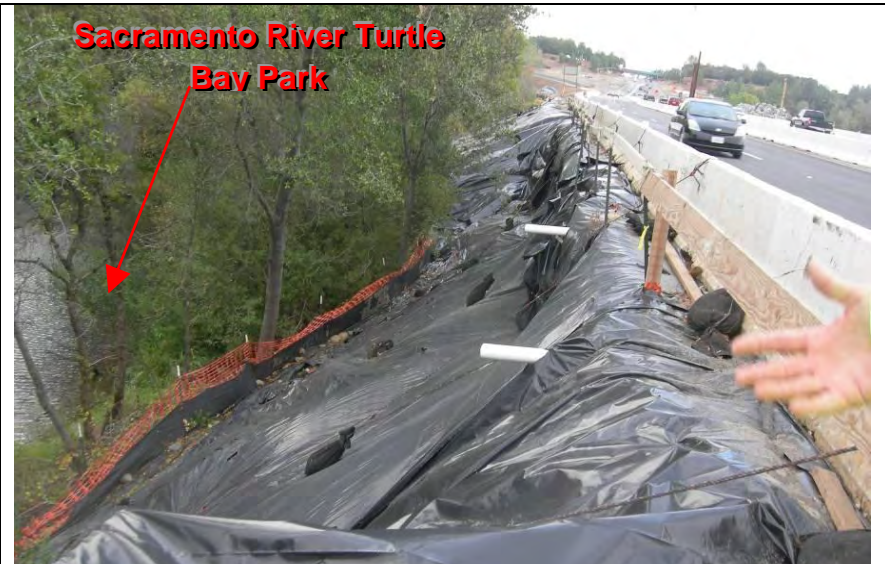
Photograph 2 – View of temporary plastic slope stabilization along the north side of I-5, at the terminus of the bike path
