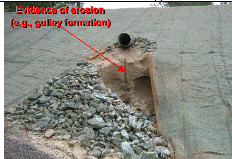
Photographs 16 – Adequate BMPs were not implemented below field constructed sediment basin No. 1 culvert outlet pipe.
