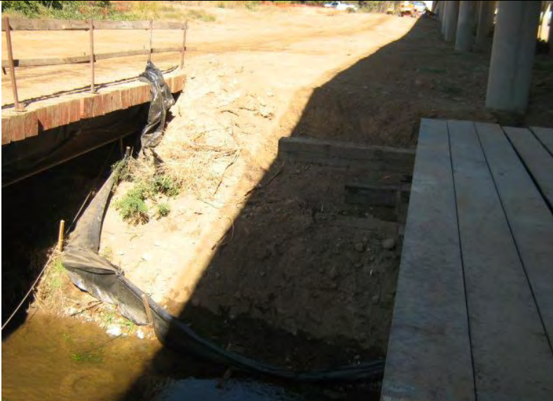
Photograph 21 – Silt Fence BMP not properly maintained (e.g., collapsed) adjacent to Yankee Slough. Note area of disturbance up-gradient.
