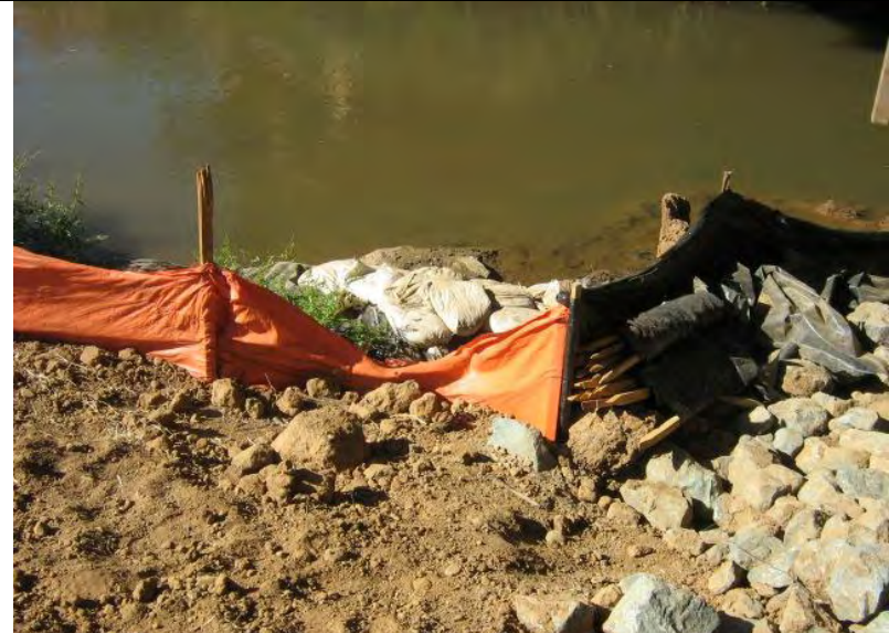
Photograph 14 – Silt Fence BMP not adequately maintained (e.g., down in areas) adjacent to Auburn Ravine
