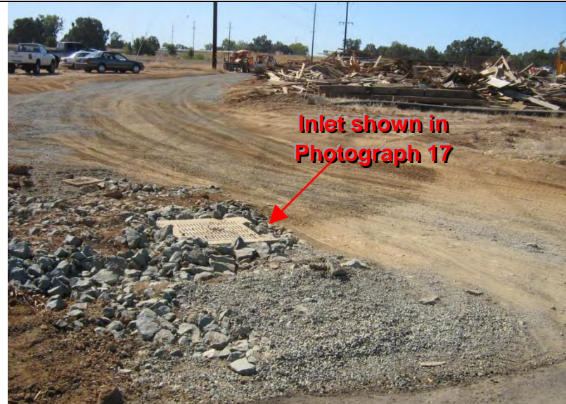
Photographs 16 – Adequate inlet protection and vehicle tracking control BMPs had not been implemented adj. to entrance off Feather River Blvd.
