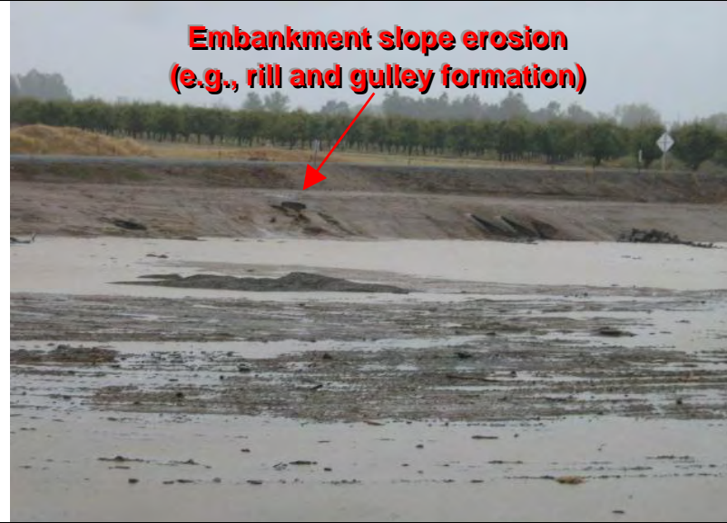
Photograph 2 – Erosion of unstabilized sediment basin and associated embankment slopes
