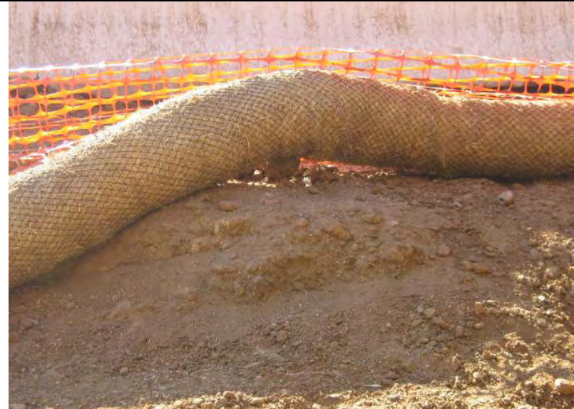
Photographs 16 – Straw wattle BMP not properly installed (e.g., not entrenched) up-gradient of Auburn Ravine
