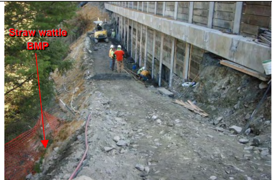
Photograph 2 – Example of straw wattle BMP implemented down-gradient of disturbance and retaining wall construction
