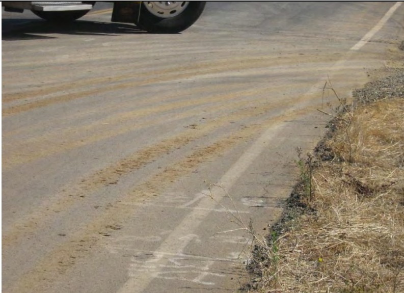
Photograph 15 – Sediment transport from areas of disturbance onto Feather River Boulevard, a public roadway.
