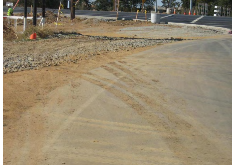
Photograph 14 – Sediment transport from areas of disturbance onto Feather River Boulevard, a public roadway.
