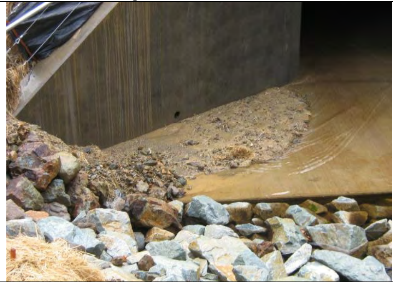
Photograph 12 – Close-up view of Photograph 11 depicting the discharge of sediment and sediment accumulation in Yankee Gulch
