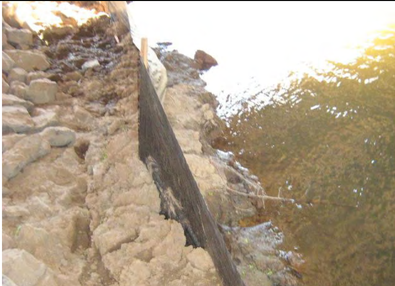
Photograph 15 – SF BMP not adequately maintained (e.g., sediment placement over ½ the effective height) adjacent to Auburn Ravine
