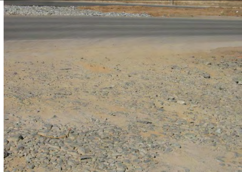
Photograph 6 – Close-up of Photograph 5 depicting sediment in VTC pad, and rock which was thin, sparse and compacted in areas
