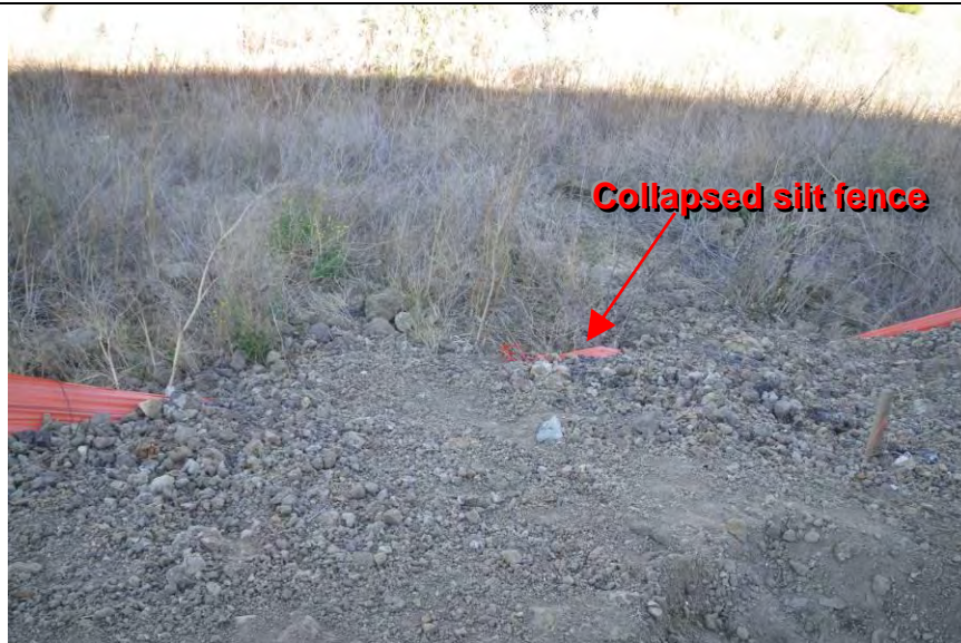
Photograph 7— Collapsed silt fence due to slide
