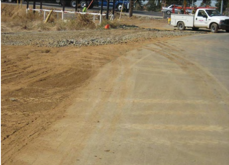
Photograph 13 – Sediment transport from areas of disturbance onto Feather River Boulevard, a public roadway.
