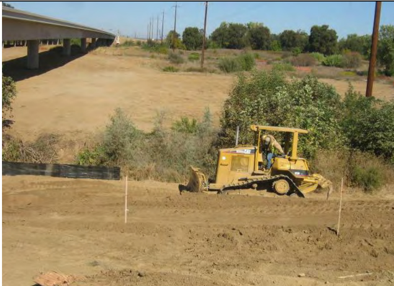
Photograph 25 – SF not adequately implemented for all land disturbing activities to prevent the discharge of sediment to Yankee Slough
