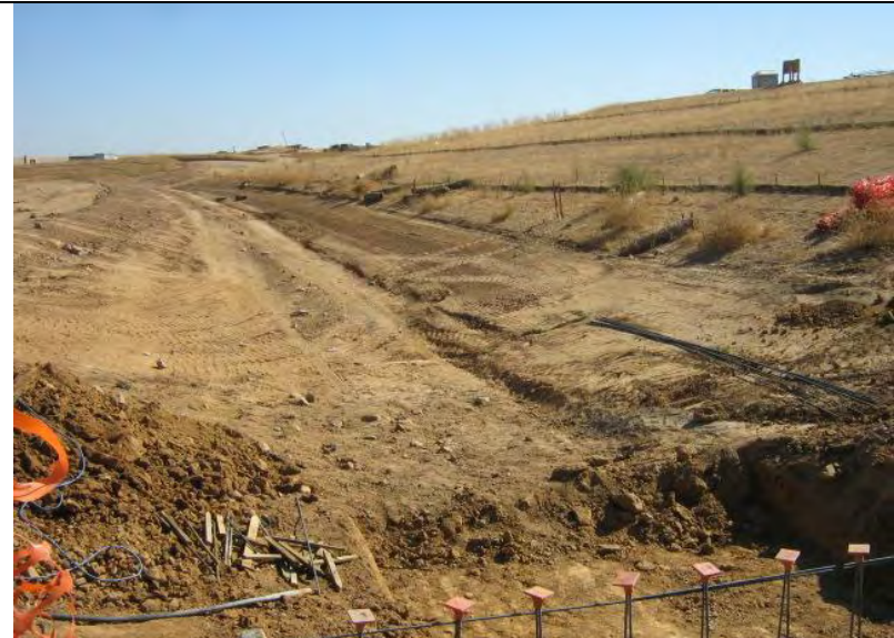
Photograph 8 – Disturbed conveyance channel with no slope run-on BMPs or erosion and sediment control BMPs near the S. Ingram Slough.
