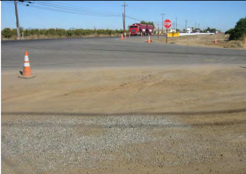
Photograph 11 –Tracking control BMPs were not implemented near Station 346 + 70.
