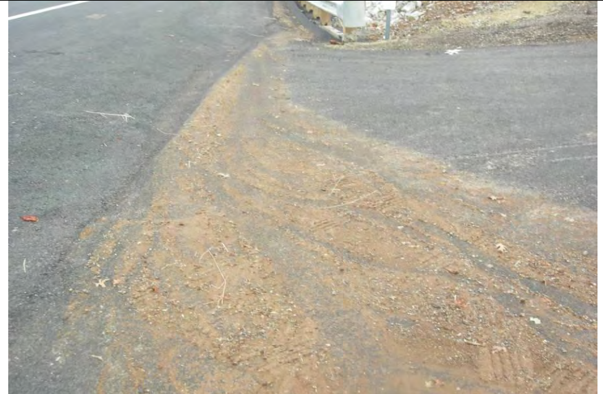
Photograph 6 – Sediment discharge along the highway from Photograph 5
