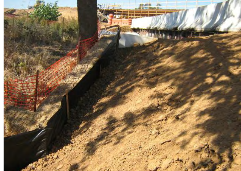
Photograph 10 – Silt fence BMPs installed backwards (e.g., stakes on the upgradient side of the fabric)
