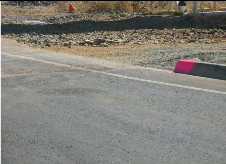
Photograph 11 – Tracking control BMPs not adequately maintained (e.g., sediment in rock pad and rock sparse in areas)
