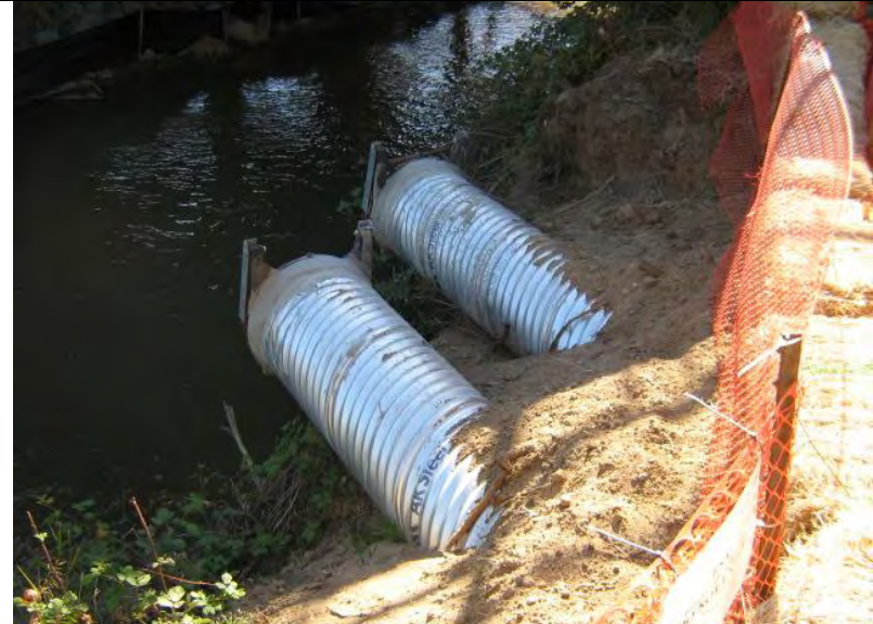
Photograph 18 – Disturbed slope area adjacent to pollution prevention BMP outlet pipes adjacent to Auburn Ravine.
