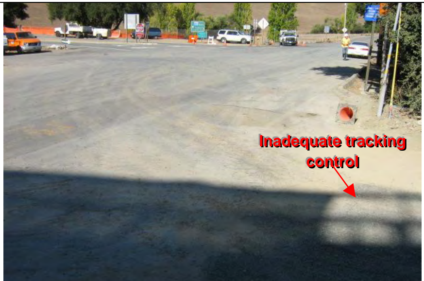
Photograph 9— Sediment conveyed onto roadway
