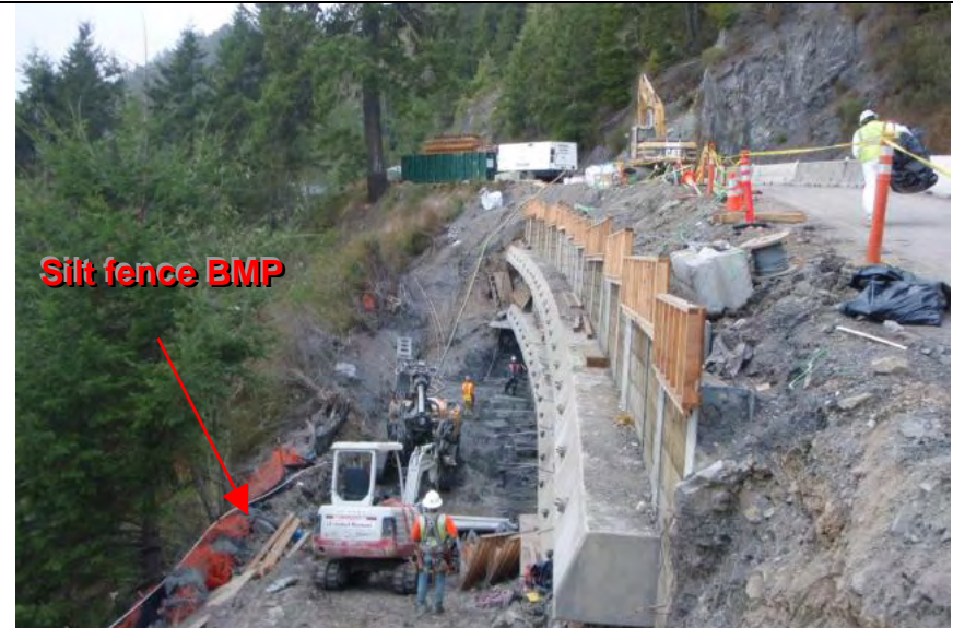
Photograph 2 – Example of silt fence BMP implemented down-gradient of disturbance and retaining wall construction
