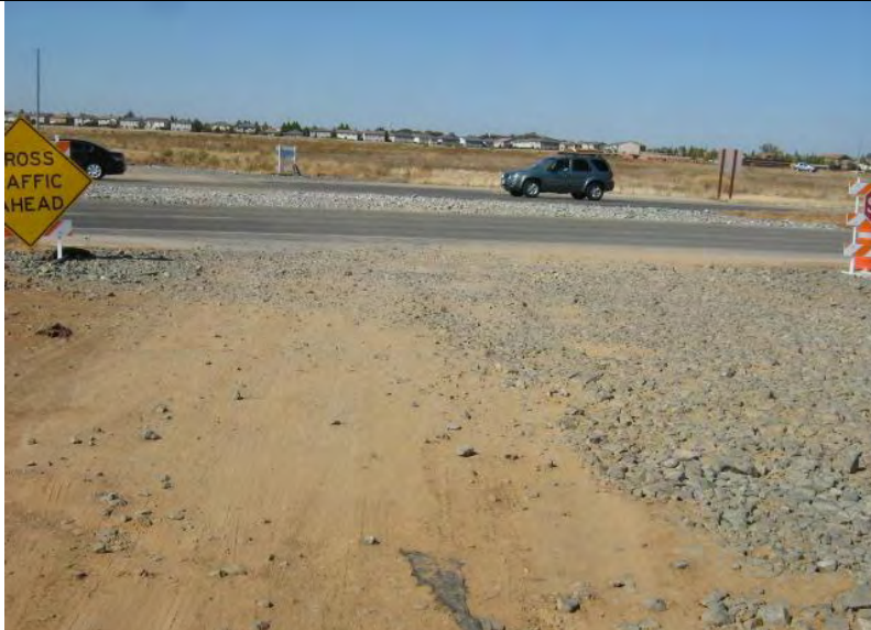
Photograph 5 – Vehicle tracking pad BMP not adequately maintained (e.g., sediment in pad, and rock thin and sparse in areas)
