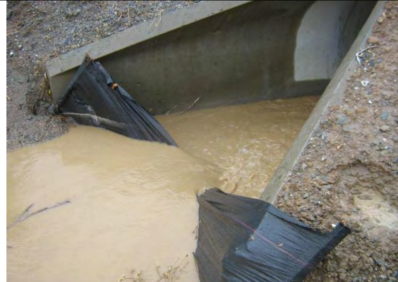
Photograph 10 – Inappropriate BMP selection (e.g., silt fence implemented in area of concentrated flow) and discharge of sediment laden runoff
