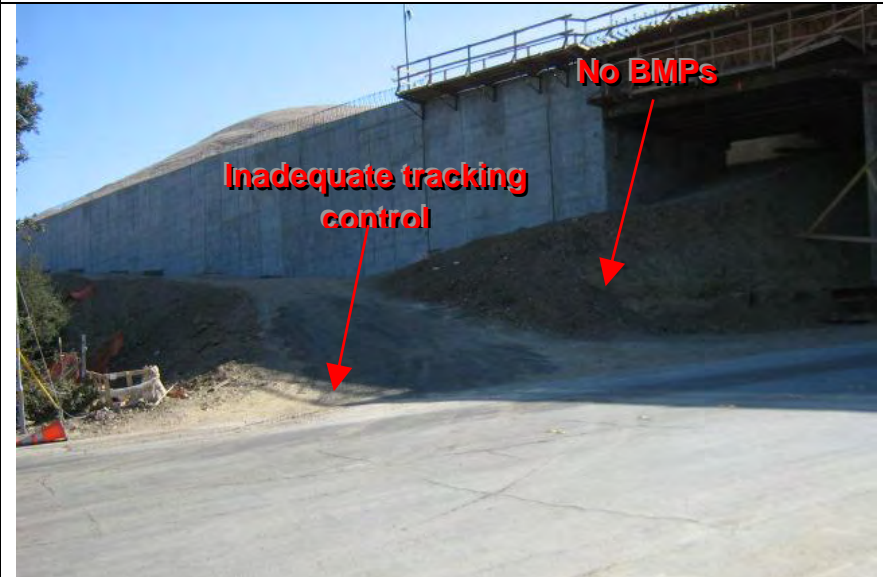
Photograph 8 – View of fill slope along access road without BMPs and vehicle tracking control pad
