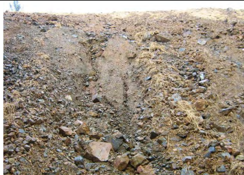
Photograph 4 – Visible evidence of erosion (e.g., rill and gully formation) on the disturbed slope area draining to Crystal Creek
