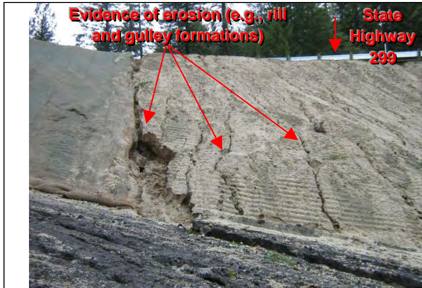
Photograph 1 – Disturbed slope areas adjacent to State Highway 299 with evidence of erosion (e.g., rill and gulley formations)
