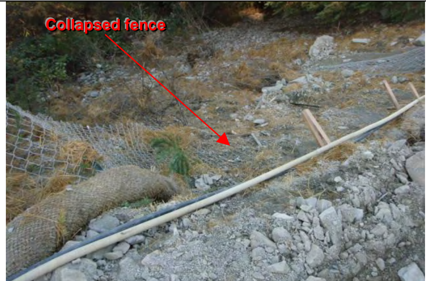
Photograph 6 – Example of collapsed section of metal fence
