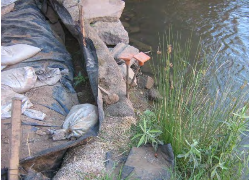
Photograph 13 – Differing vantage point from Photograph 12 depicting unmaintained Silt Fence BMP adjacent to Auburn Ravine
