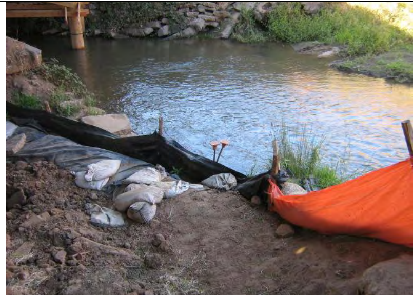
Photograph 12 – Silt Fence BMP not adequately maintained (e.g., down in areas; deteriorated) adjacent to Auburn Ravine
