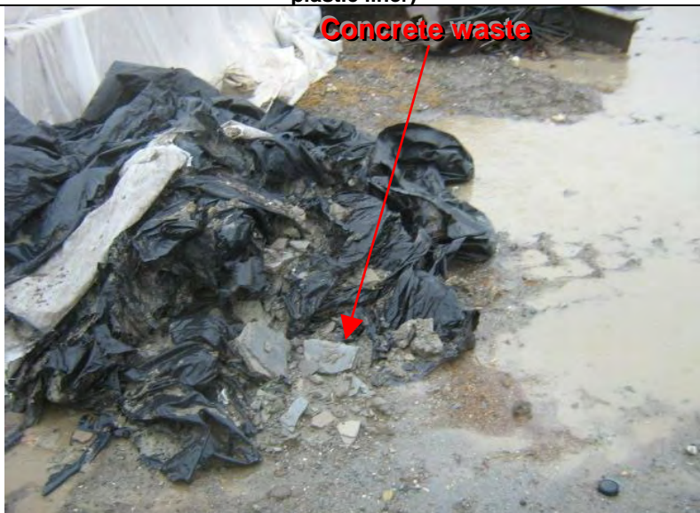
Photograph 3 – Concrete waste on the ground surface directly adjacent to the concrete washout
