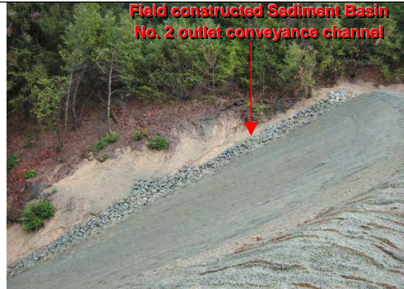
Photograph 4 – Vantage point of the outlet conveyance channel for the field constructed sediment basin No. 2
