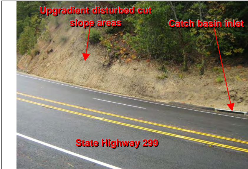
Photograph 21—BMPs were not implemented to prevent the discharge of sediment from up-gradient disturbed cut slope areas to catch basin inlets.
