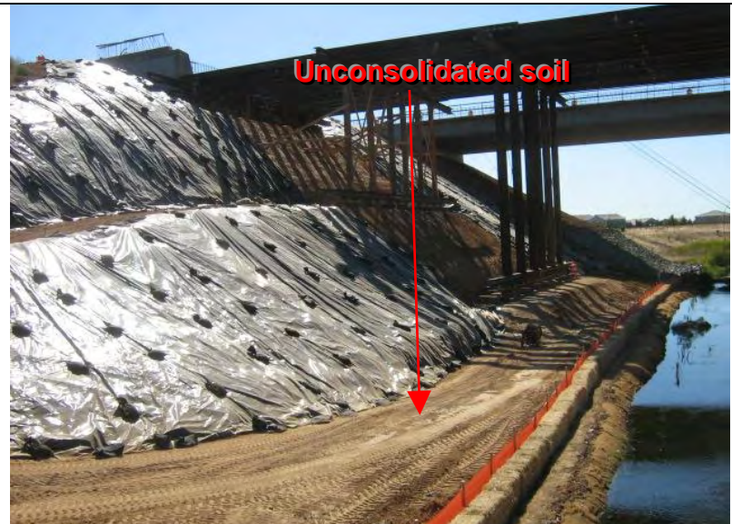
Photograph 4 – No BMPs to control concentrated flow off of the plastic and across the unconsolidated material at the toe of the slope
