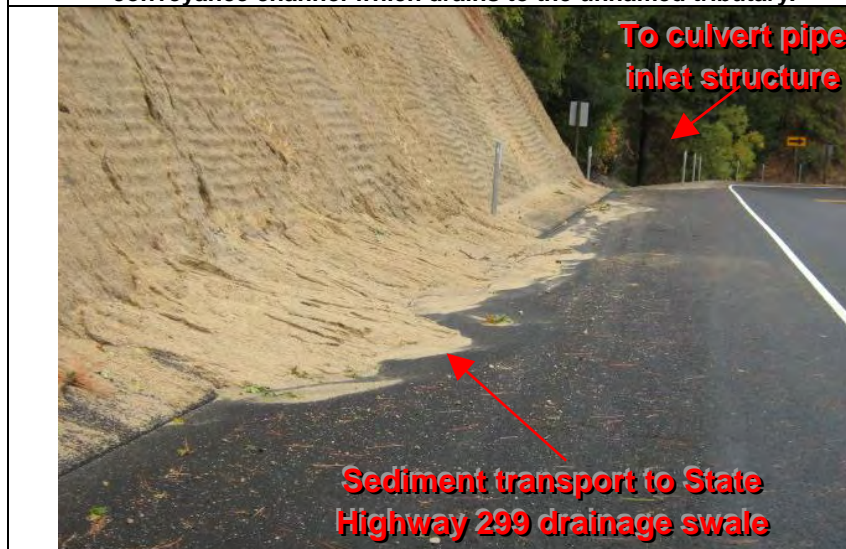
Photograph 19—Evidence of sediment transport to State Highway 299 drainage swale from the adjacent unstabilized disturbed cut slope area.
