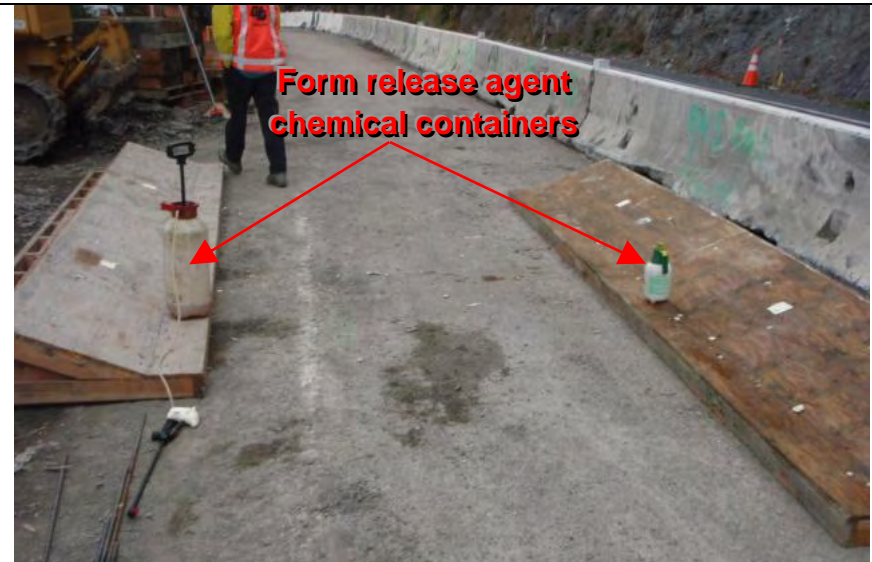
Photograph 10— Chemical sprayers not within secondary containment
