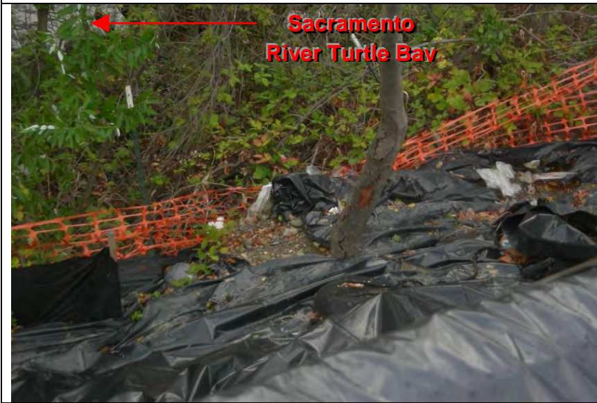
Photograph 3 – View of deteriorated slope stabilization BMP and collapsed silt fence in Photograph 2
