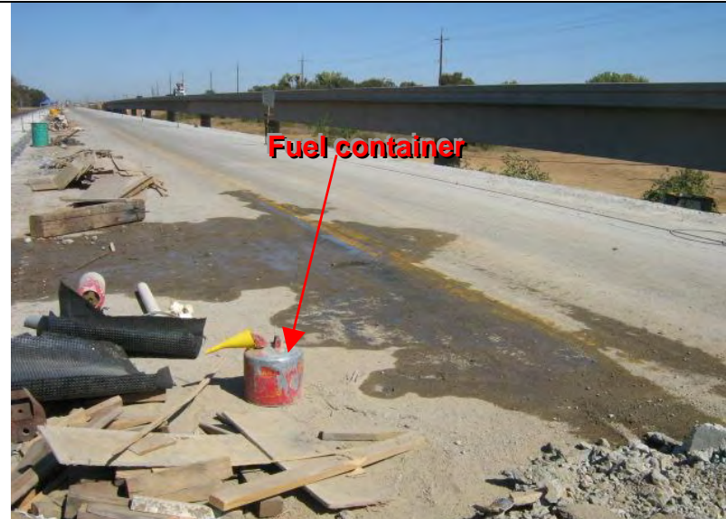
Photograph 18 – Inadequate materials handling and storage
