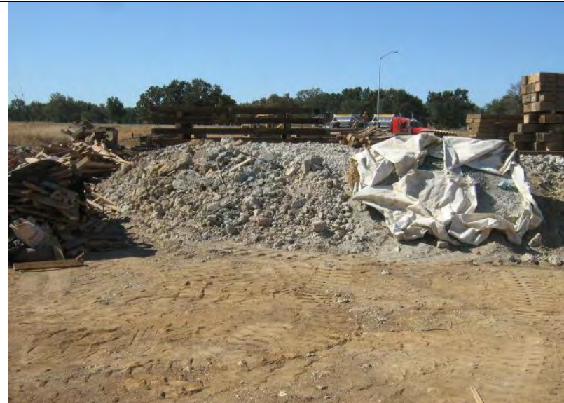
Photograph 8 – Uncontrolled/uncontained concrete waste
