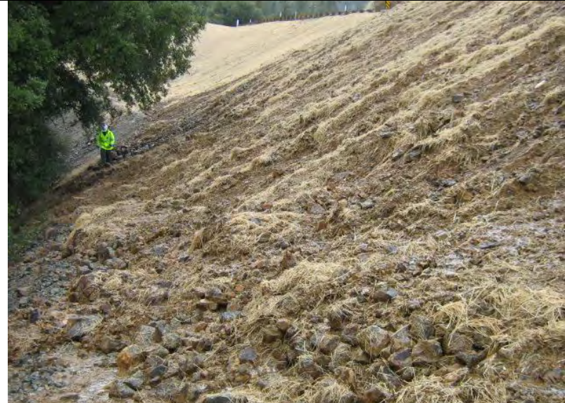
Photograph 2 – Evidence of erosion and slope failure on disturbed slope areas draining to Crystal Creek on the south side of State Highway 299
