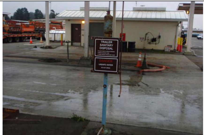
Photograph 2 – Another view of covered wash rack
