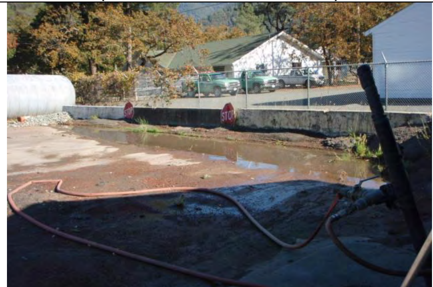
Photograph 12 – Bermed area used for truck bed washing
