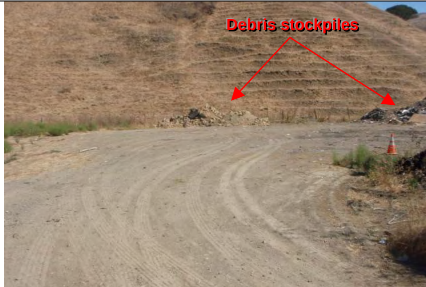
Photograph 1 – Entrance to temporary storage site
