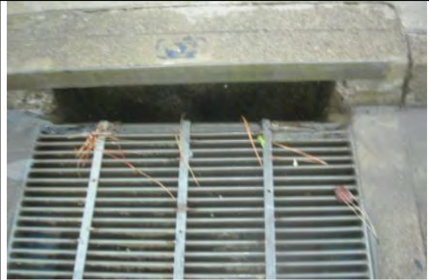
Photograph 2 – Storm drain from Photograph 1
