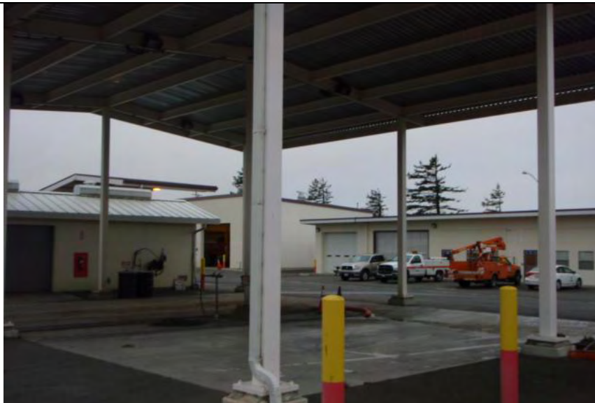
Photograph 1 – Covered wash rack
