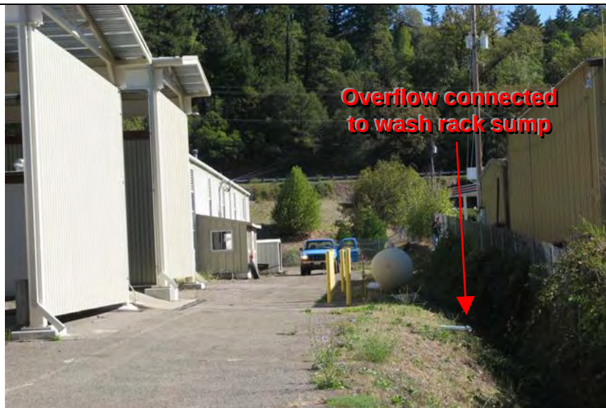
Photograph 3 – Sump overflow leading to drainage ditch
