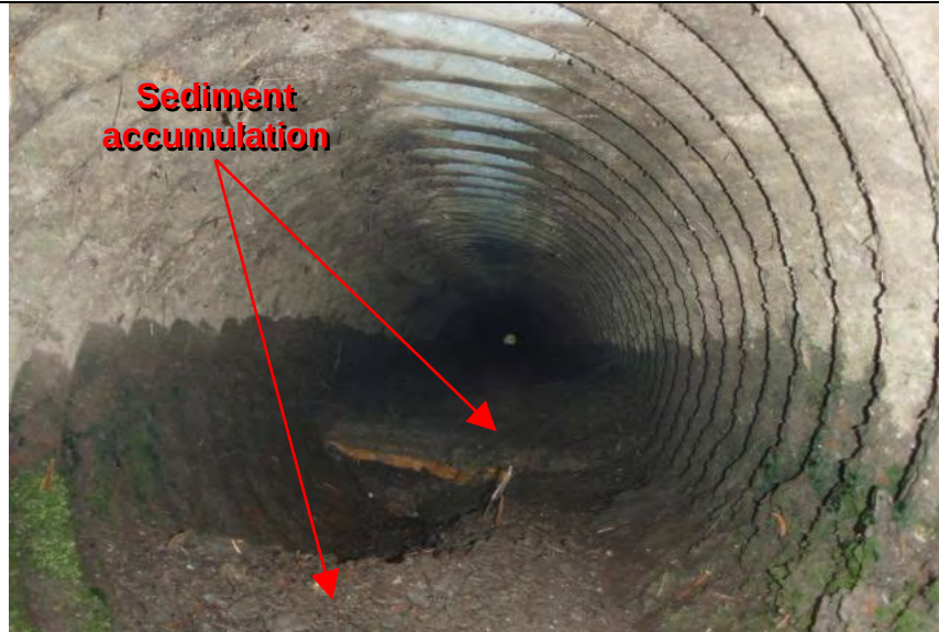
Photograph 5— View into storm drain pipe from outlet
