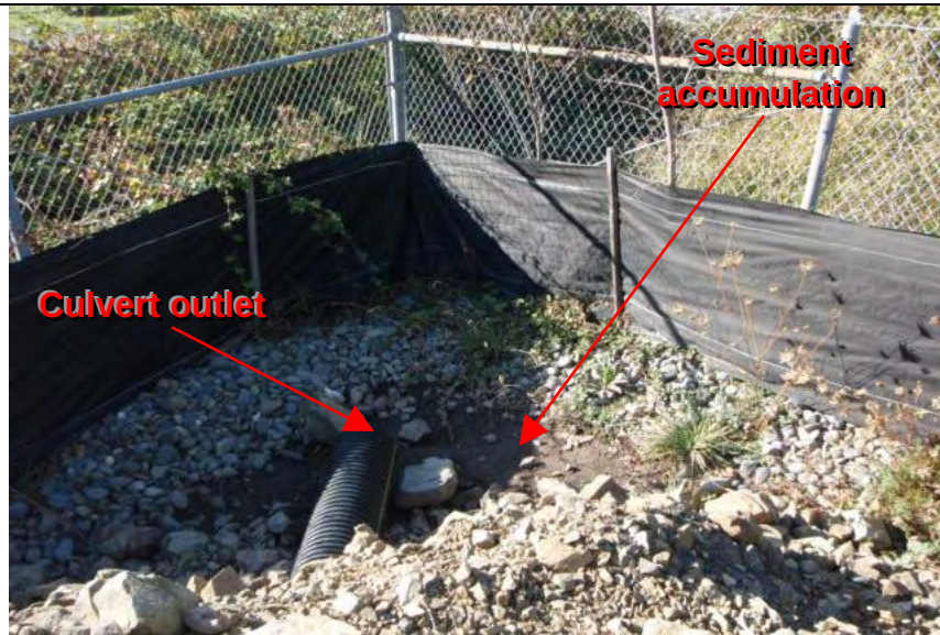
Photograph 3 – Culvert outlet to northwest corner of facility (Note: Silt fence BMP installed backwards)
