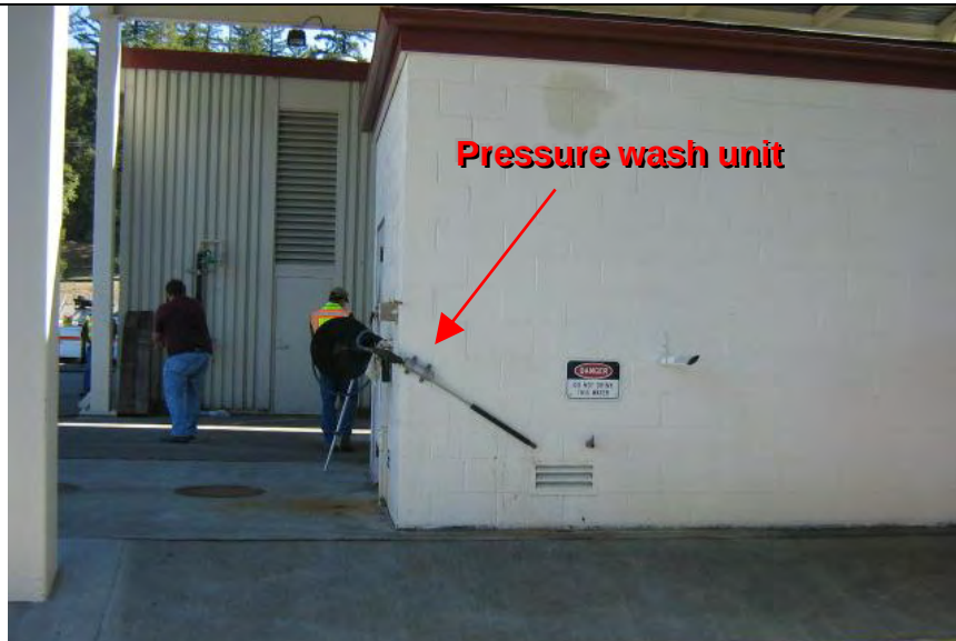
Photograph 1 – Covered wash rack
