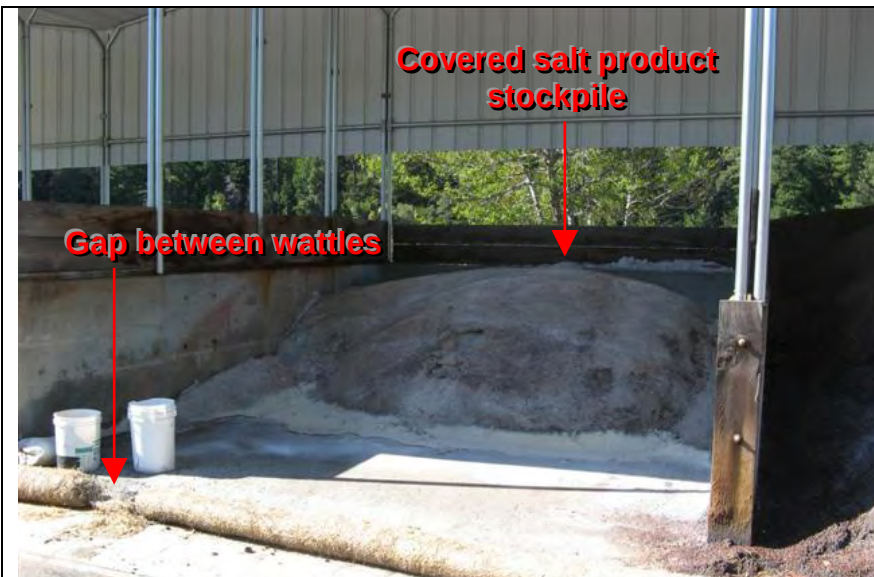
Photograph 9— Inappropriate application of wattles
