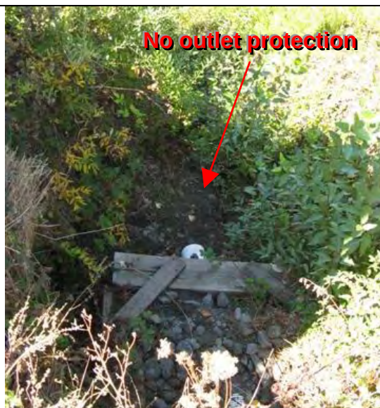
Photograph 11— Outlet pipe down-gradient of facility outfall
