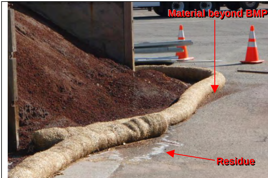
Photograph 9— Closer view of straw wattles implemented at edge of covered storage area
