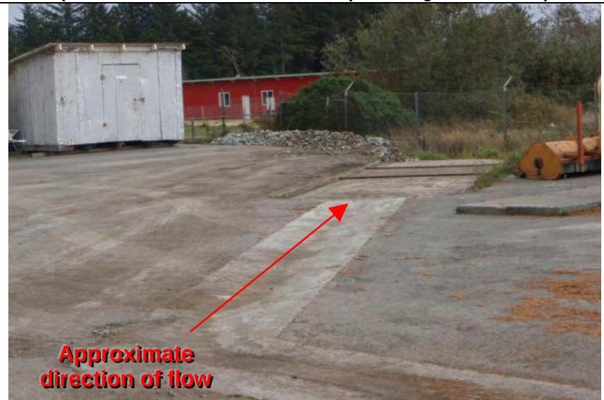
Photograph 8 – View of surface drainage system through stockpile area
