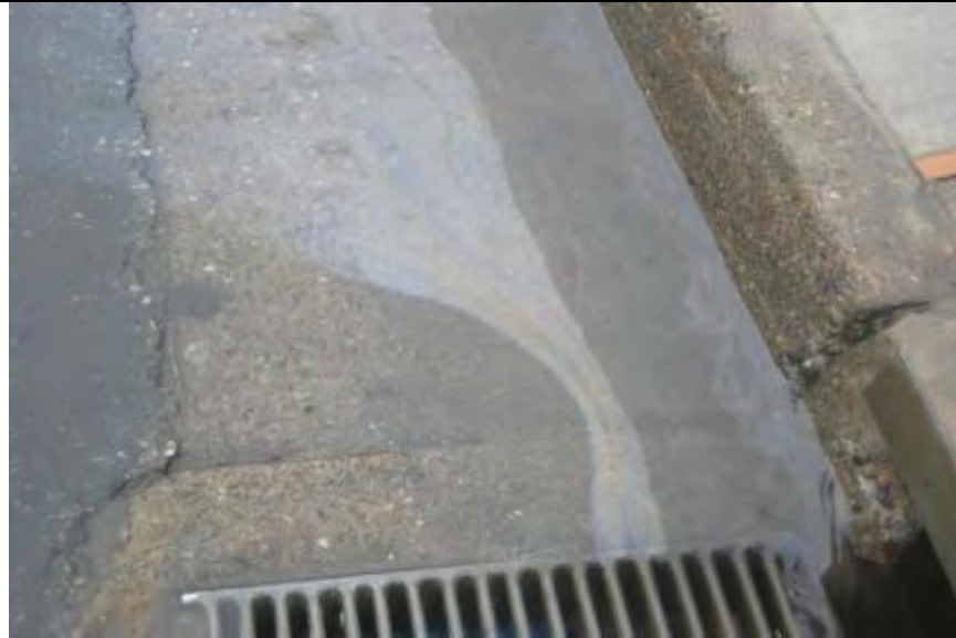
Photograph 1 – Visible sheen entering storm drain
