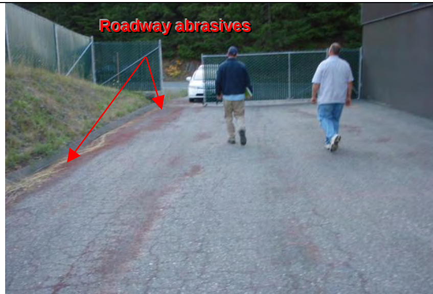
Photograph 6 – Roadway abrasives on impervious ground surface
