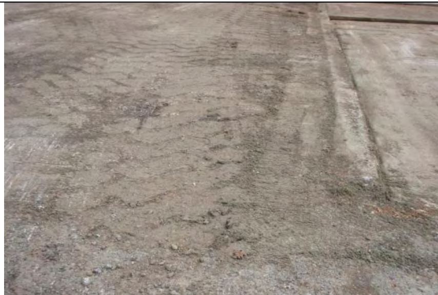
Photograph 7— Closer view of sediment accumulation on impervious ground surface
