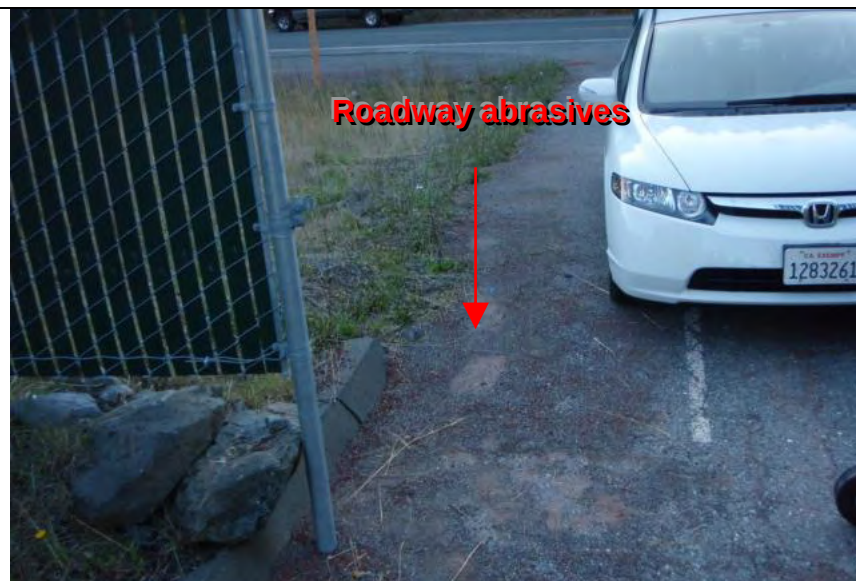
Photograph 7— Roadway abrasives outside facility entrance
