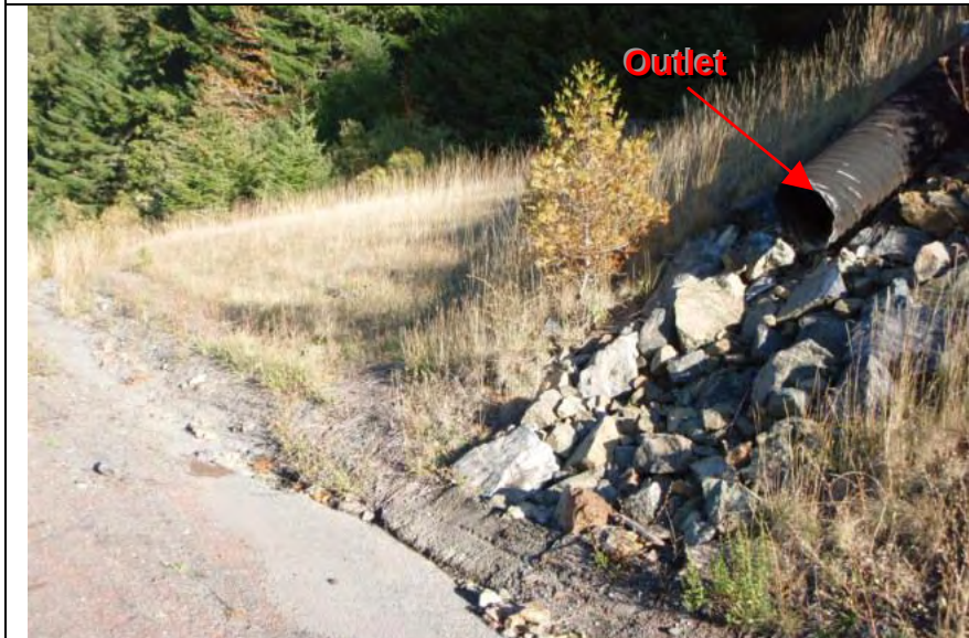
Photograph 3 – Discharge location from inlet shown in Photograph 2
