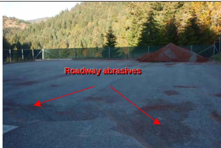
Photograph 5— Roadway abrasives on impervious ground surface
