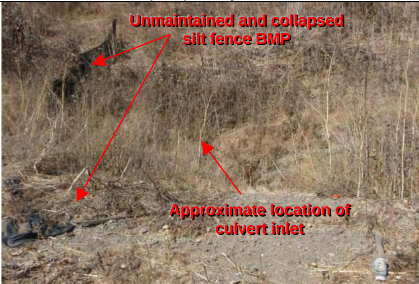
Photograph 7 – Location of culvert inlet and unmaintained and collapsed silt fence BMP up-gradient of inlet
