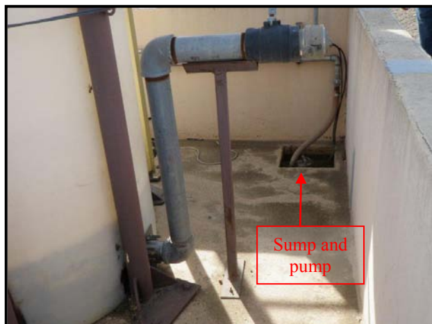
P-9: Pump-out connection used to remove the contents from the 90-day hazardous waste storage tank. Note: The sump has a pump which is used to transfer any fluid which may accumulate from rainfall events into the P-9 leachate collection tank.
