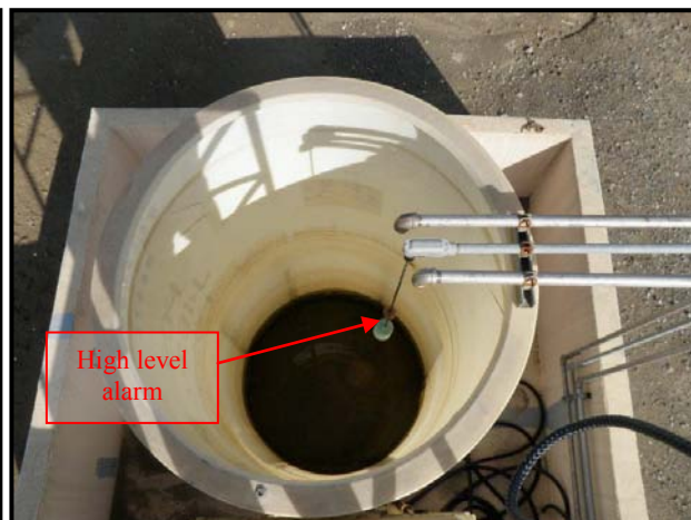
The leachate collection tank at P-9 is an open-top tank. Three pipes are located on top of the tank. One pipe is from the P-9 riser assembly, one pipe is from the P-9 tank sump, and the middle pipe is the high level alarm which ensures that the two-foot freeboard is maintained. The inspectors observed several inches of rainwater on the bottom of the tank, as described on the label.
