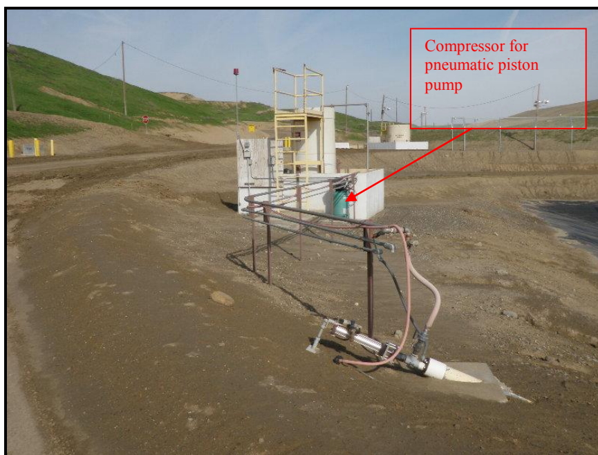
P-9: Riser assembly in the foreground leading to the leachate collection tank (facing north). A pneumatic piston pump is used to pump out the leachate sump.
