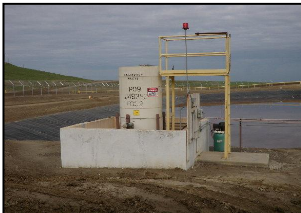
P-9: Leachate Collection Tank (facing east). Note: The panel on the right side contains the high level alarm and the magnehelic device used for determining the sump liquid level.
