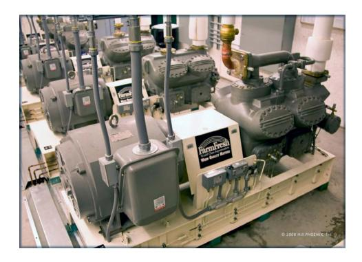
"With laser alignment, we're able to get a finer tolerance in lining up the compressors and motors and that means less vibration and energy consumption," Perry explains. "With less
