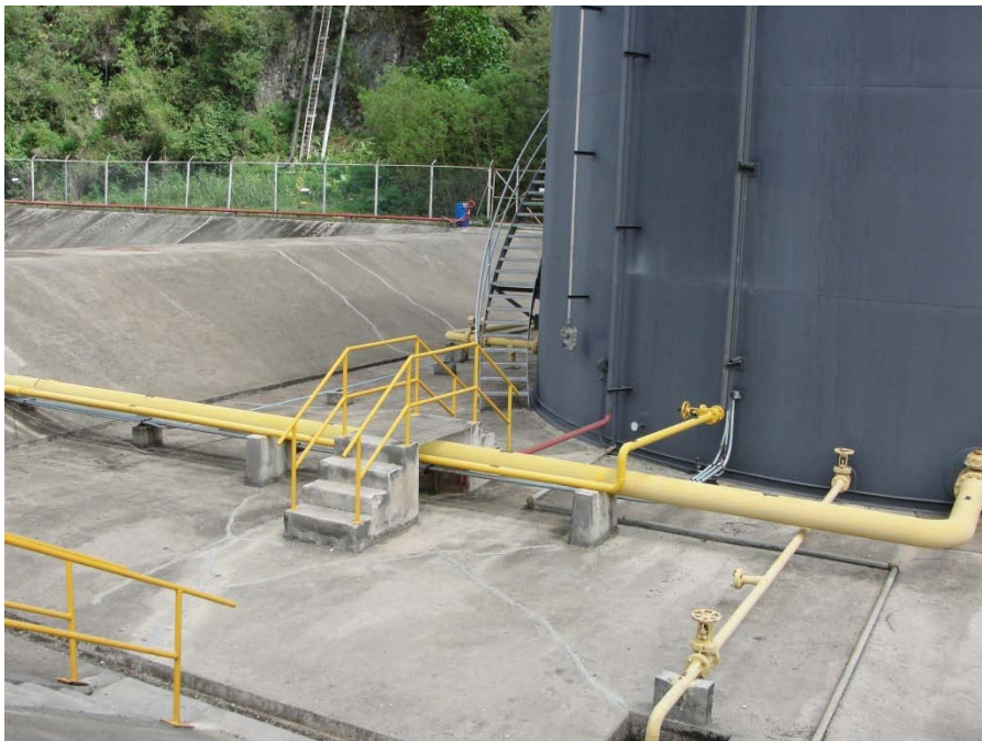
Photo 14: Secondary containment for above ground storage tanks.
