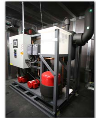
SNPS Medium Temp Pump Stations
