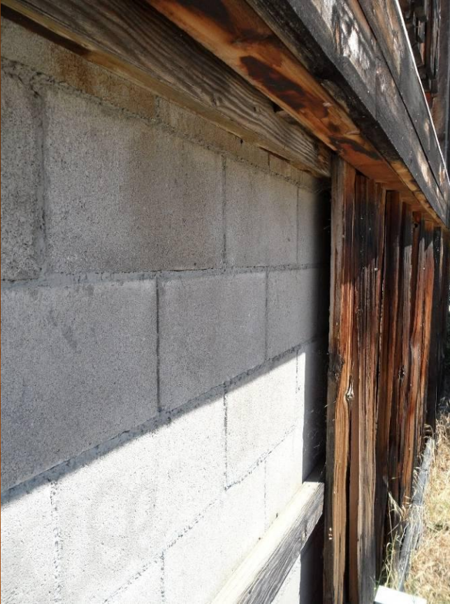
Filled concrete blocks and furring strips
