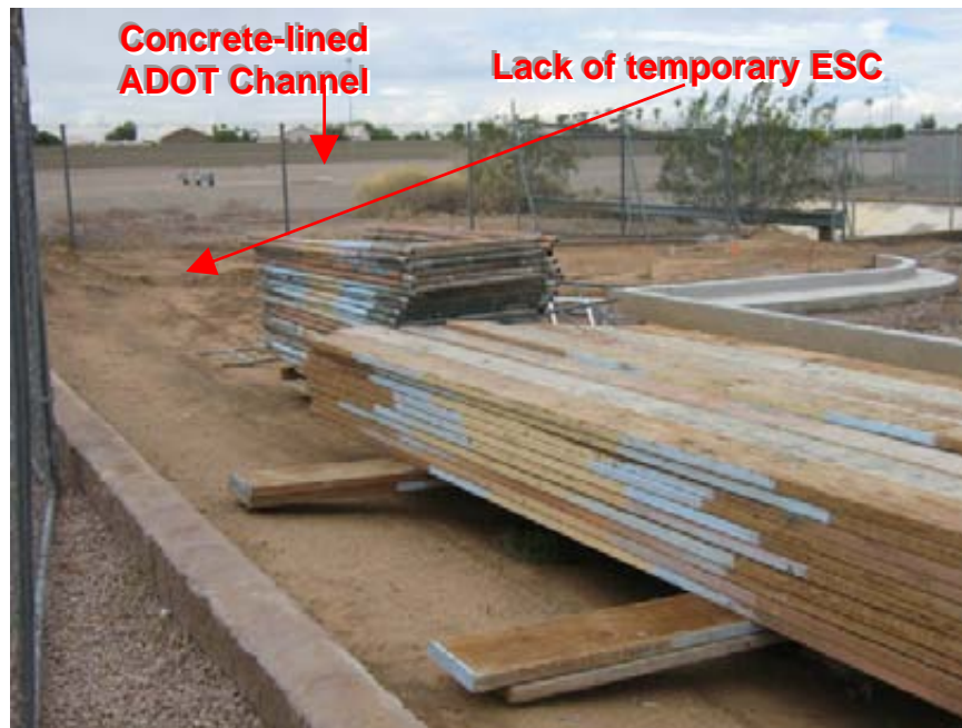
Photograph 11: Superstition Springs Commerce Center View showing proximity of site to the ADOT Channel and lack of BMPs
