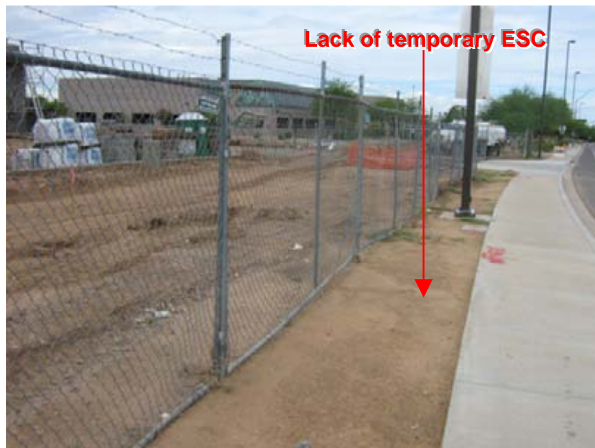
Photograph 12: Superstition Springs Commerce Center BMPs were not implemented as perimeter control along Hampton Avenue, between the disturbed area and the offsite curb and gutter flowline
