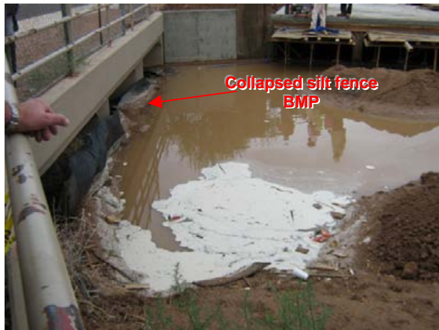
Photograph 6: Mountain View Village Center Collapsed silt fence BMP installed within the concentrated flow of the drainage channel prior to exiting the site
