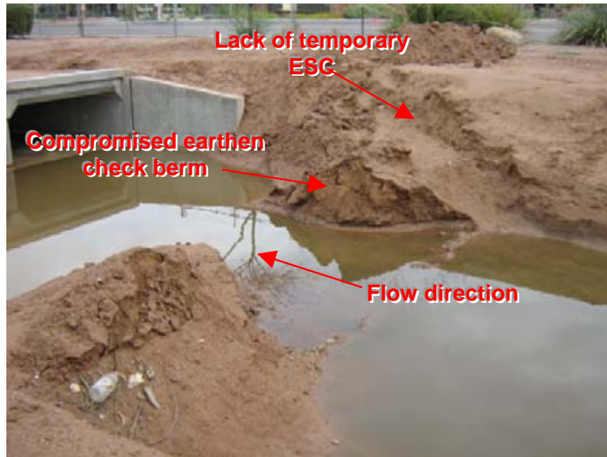
Photograph 3: Mountain View Village Center Earthen check berm consisting of unconsolidated fill had been placed within the drainage channel and was compromised by a recent flow event
