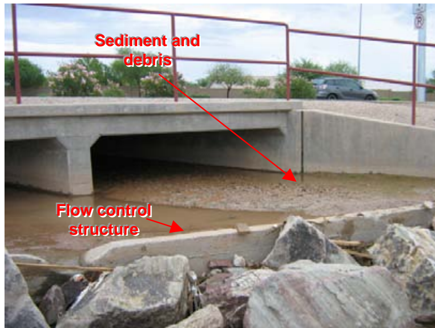
Photograph 9: Mountain View Village Center View of sediment deposition on the opposite side of the failed silt fence shown in Photograph 6
