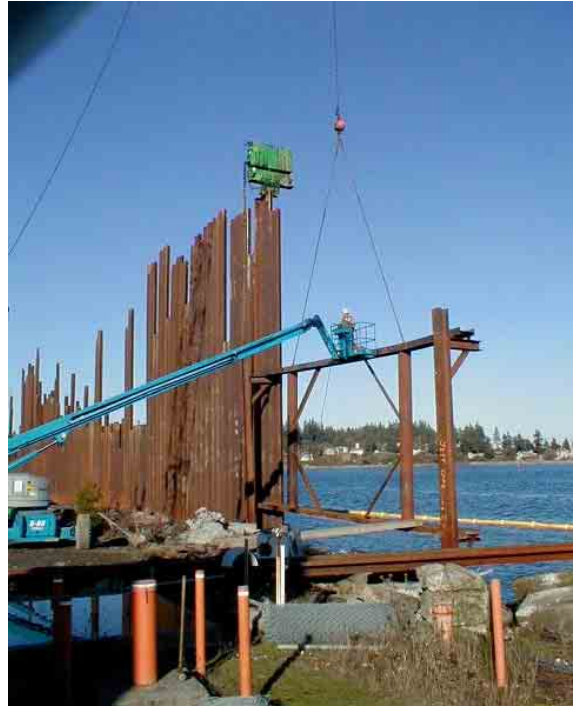
Sheet piling will be used to contain sediment
