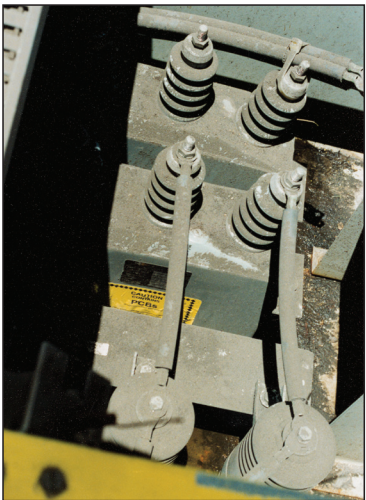
PCB Capacitors in a mine power center
