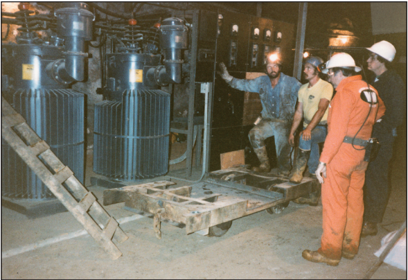
76 gallon PCB (Pyranol) transformers (cylindrical objects with cooling fins and PCB marks) on the 20 level in the Eagle Mine at Gilman, Colorado during EPA removal due to flooding and abandonment.
