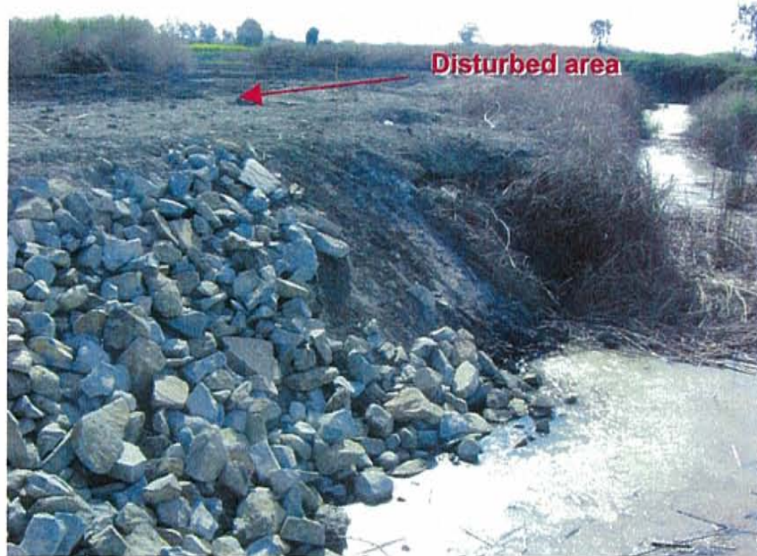
Photograph 7: BMPs were not implemented between the disturbed area on the northeast side of the railway crossing and the adjacent unnamed waterway.
