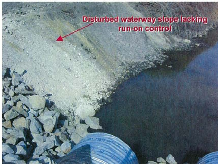
Photograph 8: Run-on control BMPs were not implemented between the disturbed area on the southwest side of the railway crossing and the adjacent unnamed waterway.
