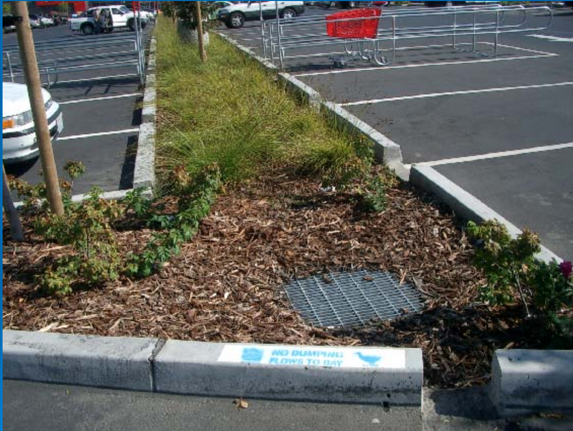
Parking lot treatment- vegetative buffer strip
