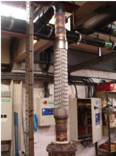
**Incorrectly installed vibration eliminator**
