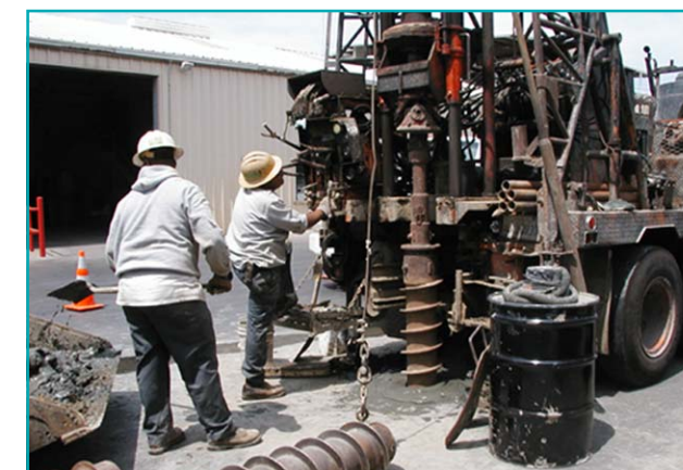
Installation of a monitoring well at Romic.
