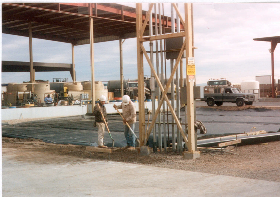
Final preparations on liner prior to covering
