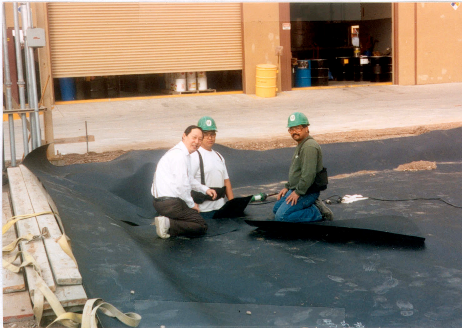
Sump area for liner being installed
