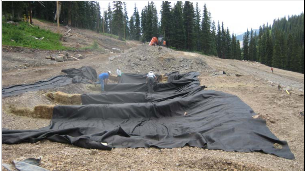
APC RETROFIT JULY 2008 – INSTALLING GEOTEXTILE ABOVE HAY BALE BERMS
