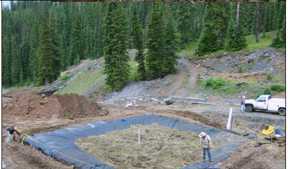
COMPLETED BCR BEING FILLED WITH MIW
