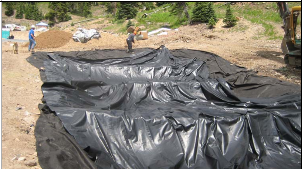
PLACING LINER ATOP GEOTEXTILE
