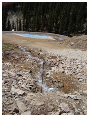
Clean Water Diversion Located East of Level 1 with a Culvert Under Road to Upper Mine
