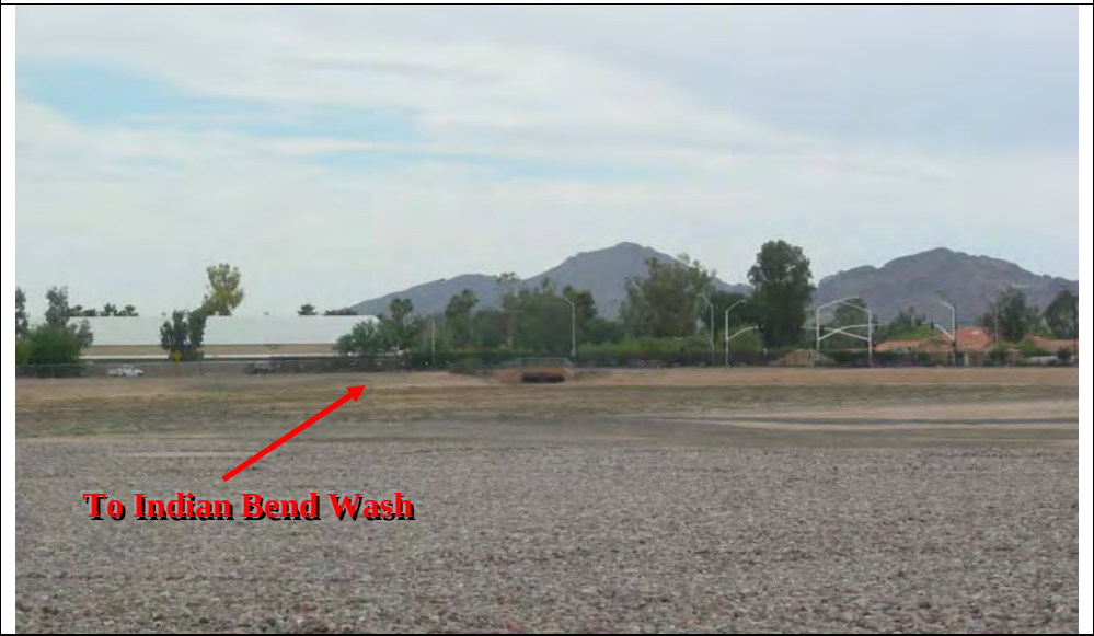
Photograph 4—View of airport detention basin, facing southeast
