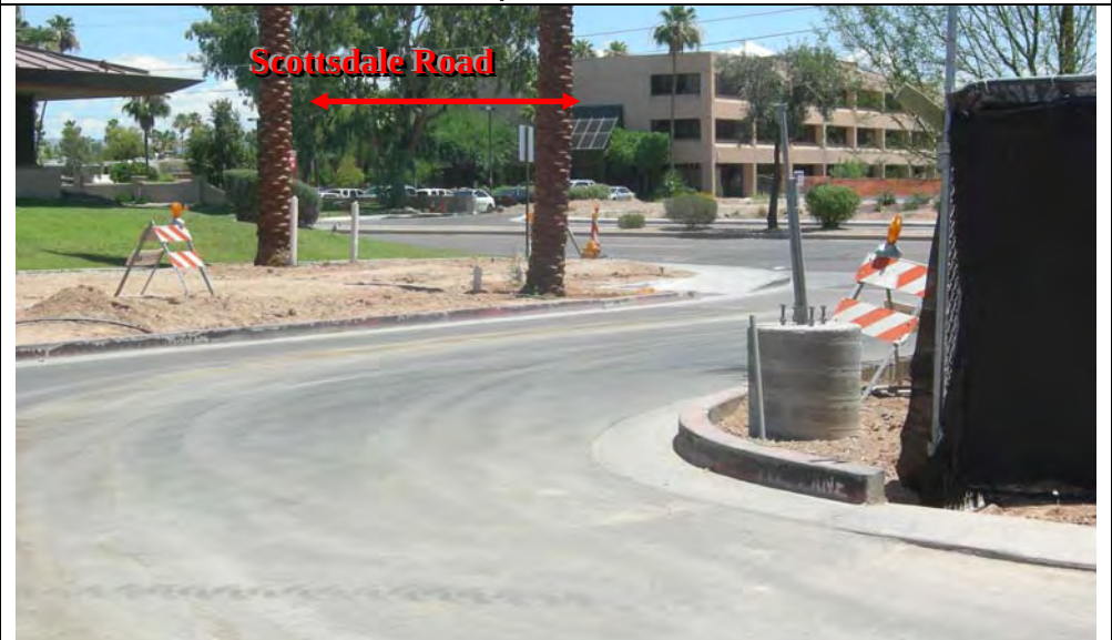
Photograph 4 – View of sediment tracking at the construction entrance at the northeast corner of the site.
