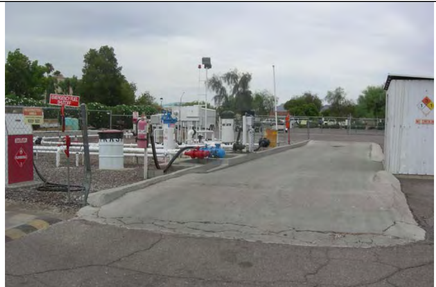
Photograph 2— View of truck fueling station
