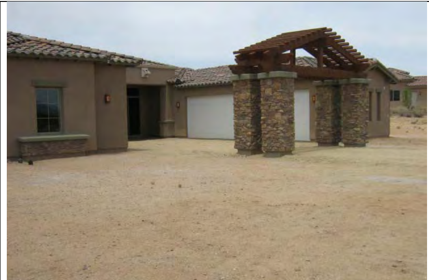
Photograph 2—Constructed home at the center of Lot 64
