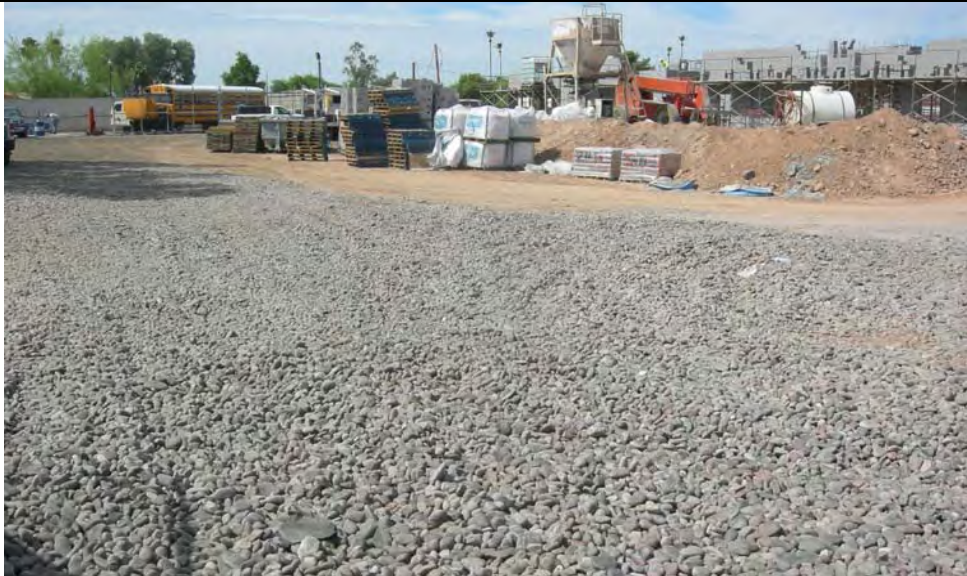
Photograph 1 – View of construction entrance facing south.
