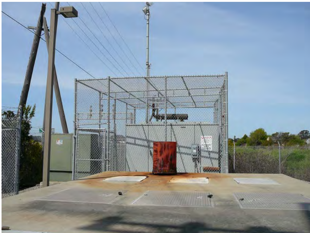
Photo 2 Generator for Burlingame pump station
