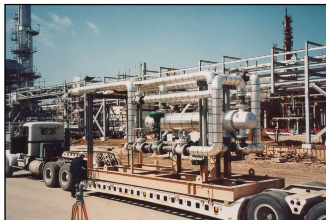
Figure 2-11 Example of a Modular Unit Arriving at a Refinery Ready for Installation
