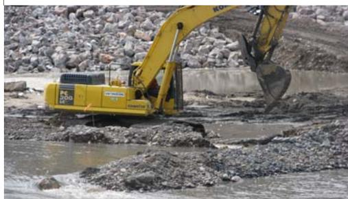
Coffer dam is breached! Clark Fork and Blackfoot Rivers begin to flow into the new channel.
