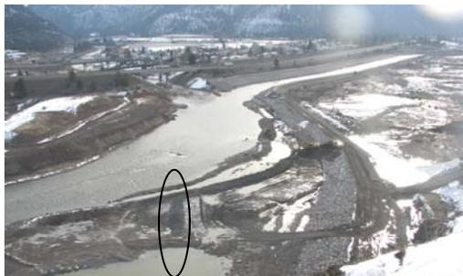
9 am: Pre-breach view of the project area. Oval shows area where coffer dam will be breached.
