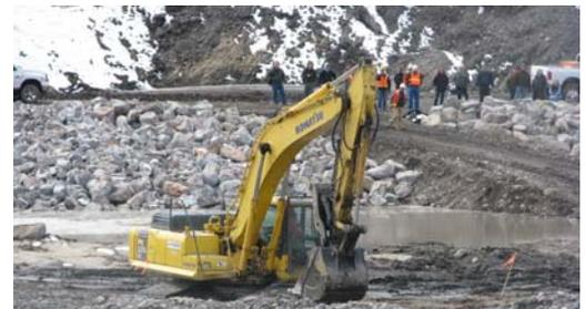
2 pm: Removing material to begin the breach of the spillway coffer dam and divert the Clark Fork and Blackfoot Rivers into the new channel
