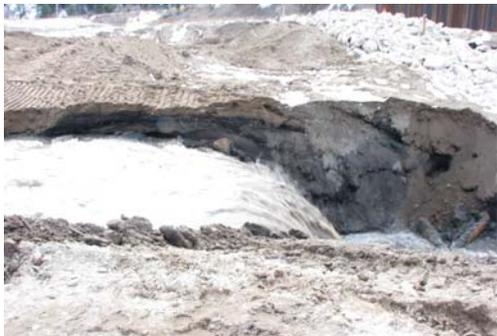
March 28, 2008: Water flowing in the breached channel. Remnants of an older coffer dam created a temporary waterfall before the timber cribbing was dislodged and the river continued to cut upstream toward the Blackfoot and Clark Fork Rivers.
