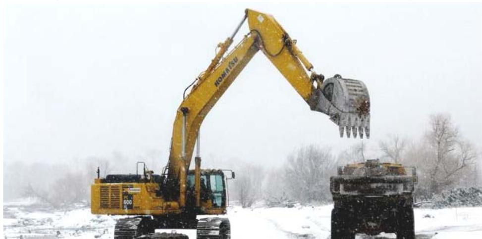
Excavating material from SAA-IV, an restoration work area upstream of the old Duck Bridge. This material serves as cover for the Tunnel Pond repository. (Photo by Mike Kustudia, CFRTAC.)
