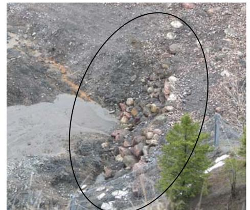
**Grade control structure as seen from the bluff.** When the de-watering pumps below the former spillway are turned off, this area will flood and the structure will no longer be visible. The "hole" is expected to fill in with cobbles and gravel during this spring's high flow.
