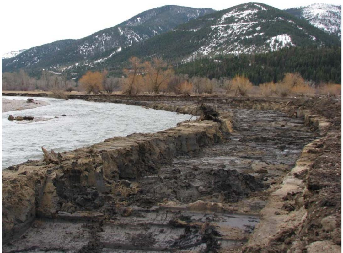
The photo above (3/3/09) shows the initial removal of contaminated sediments upstream of the remedial project area (Area 4) to prevent them from scouring during spring high flows. Preventative measures such as these reduce downstream river and fisheries impacts. If all goes as planned, up to 100,000 tons of material could be removed by April 2009.
