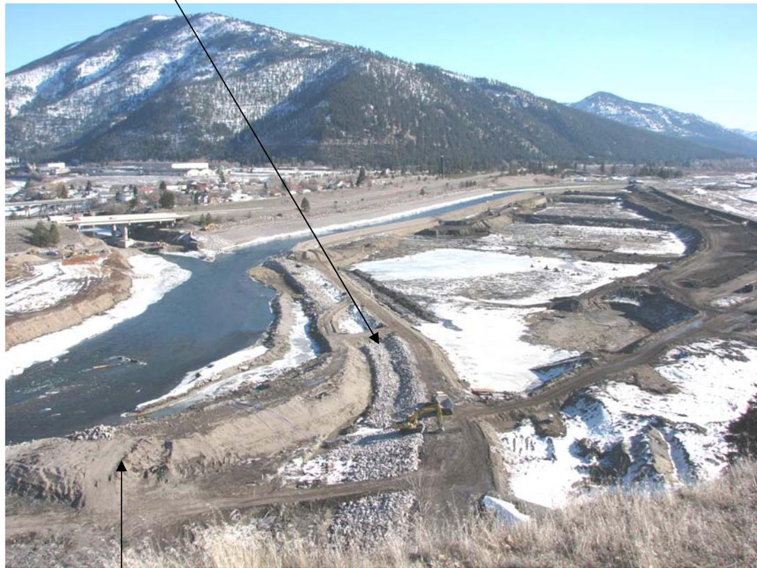
Spillway coffer dam that will be breached in March 2009. At that point, the joint Clark Fork and Blackfoot River channel will flow along the base of the Milltown bluff (not visible from this view). Much of the material on the far side of the spillway area (including portions of the divider block) will be removed before high flow this spring. Photo taken 2/3/09.
