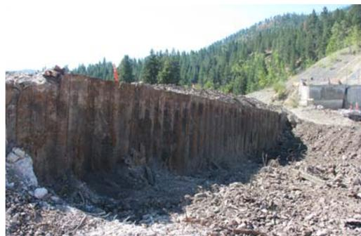
View of excavated dam spillway, 8/5. Note exposed sheet piling on upstream side of former dam.
