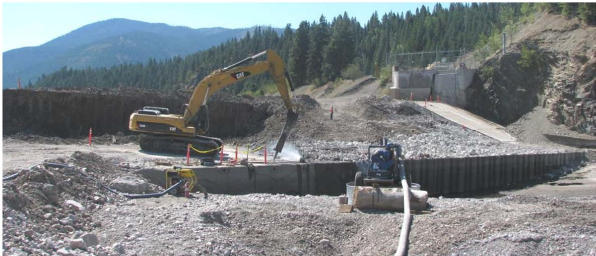
Workers are installing rock fall protection this week to safeguard workers during removal of the left (south) abutment of the former Milltown Dam. Project personnel will be working right next to the bluff. For safety reasons, the Milltown bluff is temporarily closed to the public, probably until mid-August. We will announce its re-opening.
