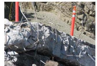
Cross-section of removed spillway concrete.
