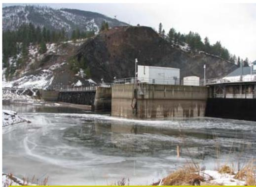
View of the Powerhouse Forebay area (views from upstream). The coffer dam would be constructed from the divider block north towards the right abutment. The coffer dam keeps the area "dry" for workers and equipment.
