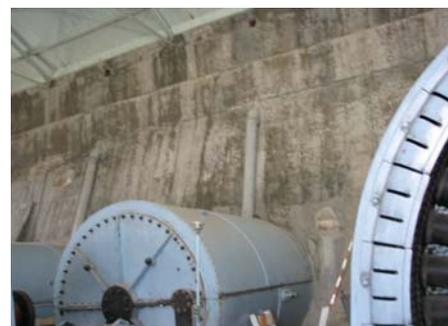
This is the now-lead paint free interior wall of the Powerhouse. Workers completed removal of the lead-based paint from this wall the Powerhouse floor.
