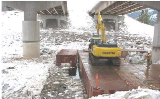
Removing barges from the Blackfoot River, 2/5/08. The 90 barges created a work platform during I-90 bridge mitigation.
