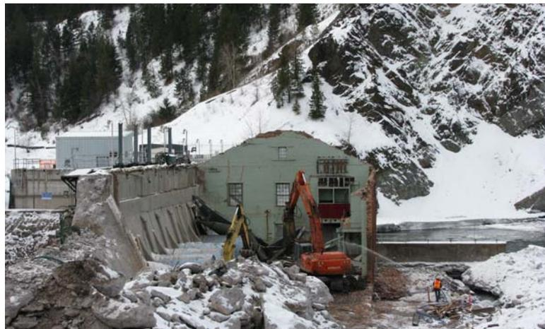
Milltown Powerhouse with north wall, part of the west wall and roof removed, 2/5/08
