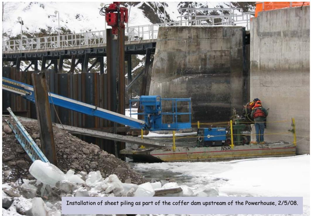
Installation of sheet piling as part of the coffer dam upstream of the Powerhouse, 2/5/08.
