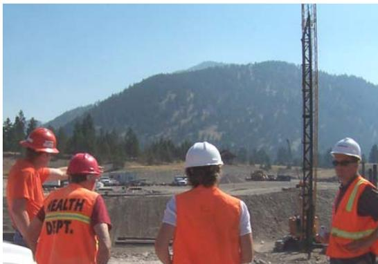
August 7: Design Review Team members tour the site and watch piles being driven into bedrock in construction of the bypass channel bridge.
