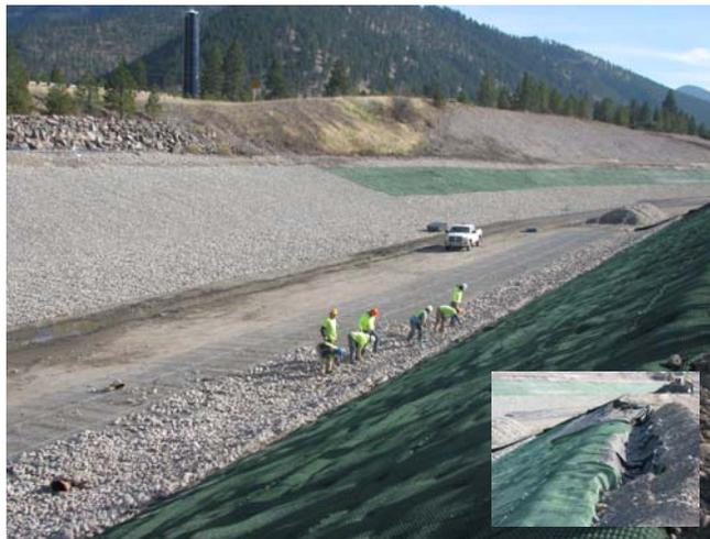
The Clark Fork River bypass channel — 4,000 feet long and built to withstand a 100-year flood event — is nearing completion. Workers are seen lining base and south side of channel. *Insert:* Anchoring the Turf Reinforcing Mat into the berm.
