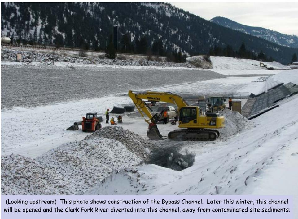
(Looking upstream) This photo shows construction of the Bypass Channel. Later this winter, this channel will be opened and the Clark Fork River diverted into this channel, away from contaminated site sediments.
