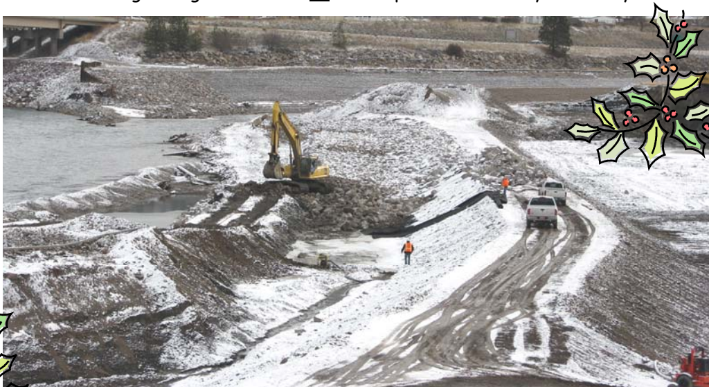
View of the flood berm along the west side of the project area. The flood berm is being strengthened to withstand a 10-year winter flow event. Photo, 12/9/08.
