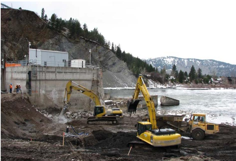
Removing the last of the right abutment of the Milltown Dam and excavating forebay (pre-dam) sediments. With the powerhouse removed, the concrete divider block is clearly visible in the background.
