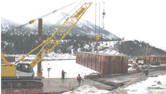
Removing barges from the Blackfoot River, 2/12/08. The 90 barges created a work platform during I-90 bridge mitigation.
