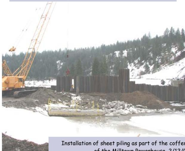
Installation of sheet piling as part of the coffer dam upstream of the Milltown Powerhouse, 2/12/08.
