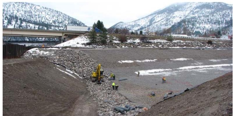
2/12/08, Tying bypass channel liner into the grade control structure at the bypass channel outlet. In a few weeks, the Clark Fork River will be diverted into this channel, isolating the river from the contaminated sediments.
