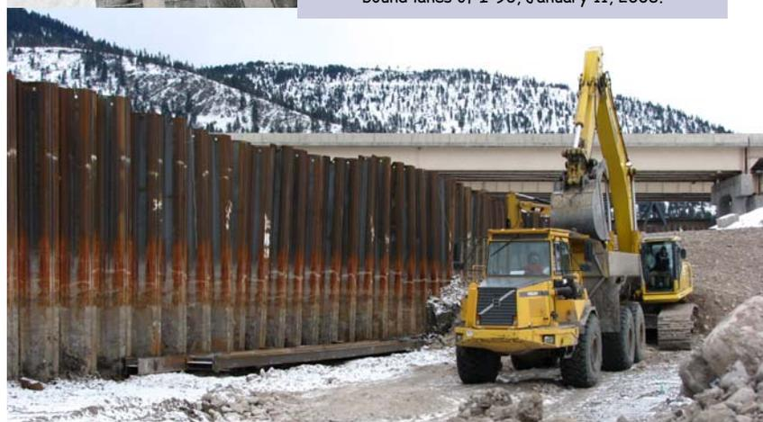
Excavation adjacent to the Sheet Piling at the Bypass Channel Outlet. Note the "walers" (metal beams) at the base of the sheet piling to provide structural support as soil is excavated away.
