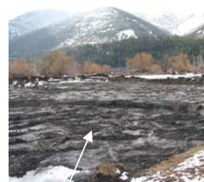
Nearly 30,000 cubic yards of sediment have been removed from upstream of old Duck Bridge. Metals levels in these sediments are only a fraction of the levels in the sediments excavated from the project area (3/17/09).
