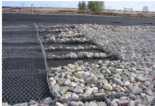
Wire cages filled with rock to form base of the reno mattress; a wire cover is then added to complete the mattress and line the Clark Fork River bypass channel.
