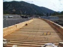
Newly constructed railroad bridge on site; ready for MRL workers to lay track, 9/18/07
