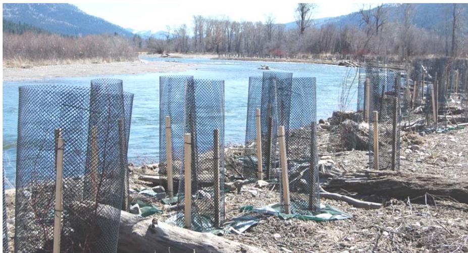
**Photo above:** View of newly planted willows along the re-constructed Clark Fork River bank in restoration area upstream of Duck Bridge.
