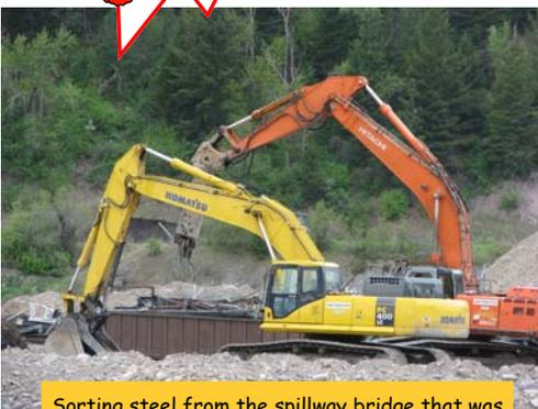
Sorting steel from the spillway bridge that was removed last week. The steel will be recycled.
