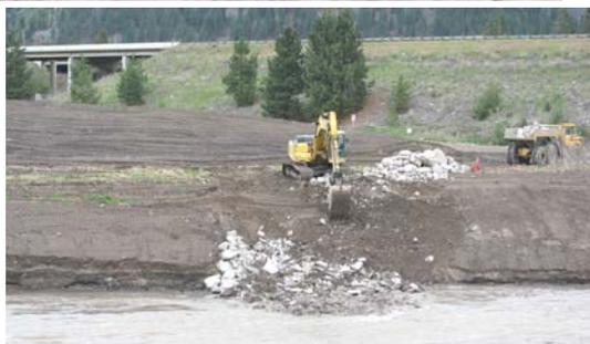
5/21/08: Building the "Flow deflector" to keep clean soils from eroding from north side of the Clark Fork River above the Dam.
