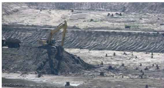
Excavating contaminated sediments unearths the pre-Reservoir Clark Fork River flood plain. Note the exposed tree stumps.
