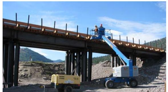
Montana Rail Link (MRL) workers installing pedestrian walkway and final touches to the on-site rail bridge over the Clark Fork River bypass channel, 9/25/07
