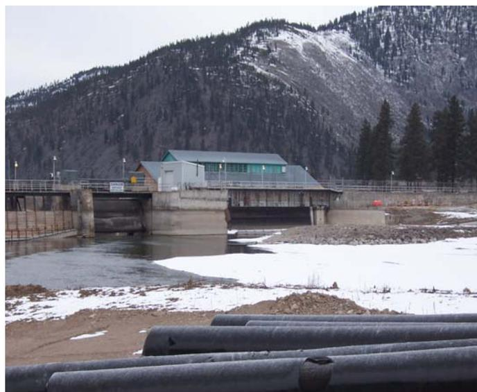
The Milltown Dam - looking downstream (west) from on top of the new Clark Fork River flood berm. In the foreground are rolls of the black geo-tech fabric used in berm construction.
