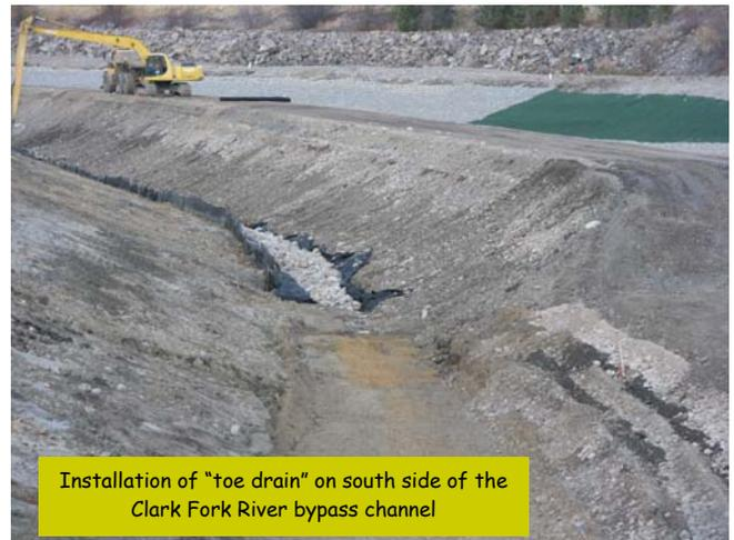
Installation of "toe drain" on south side of the Clark Fork River bypass channel
